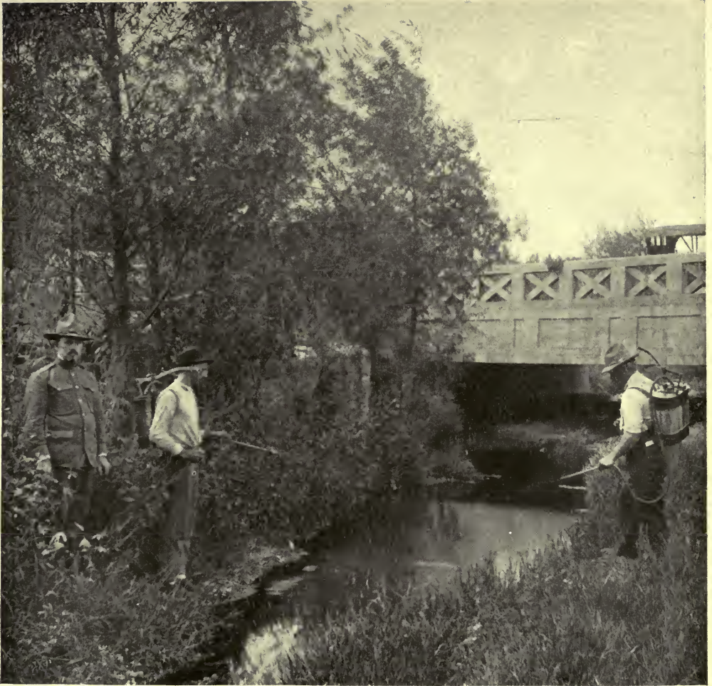
VIEW SHOWING OILING OPERATIONS FOR THE CONTROL OF MOSQUITO BREEDING
