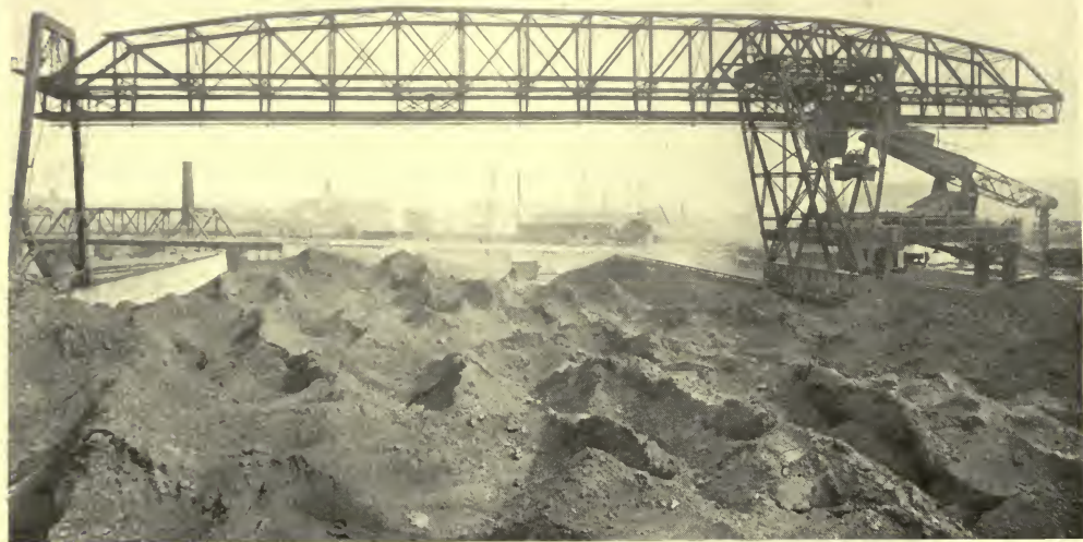
AN ORE STOCK PILE AND HANDLING MACHINERY: CLEVELAND, OHIO
