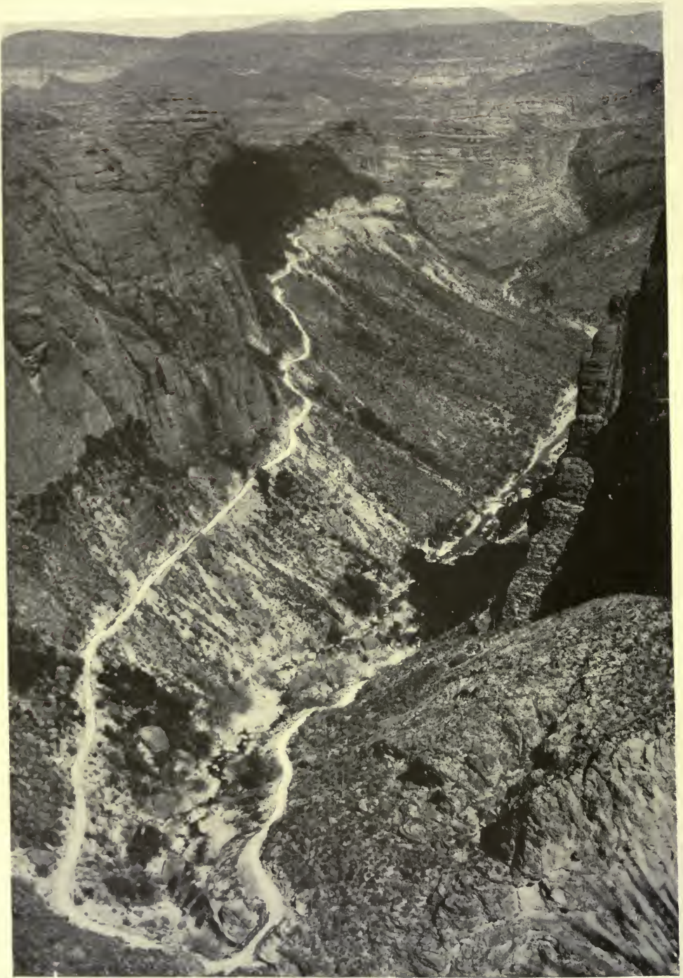
THE EAST, WEST, NORTH, AND SOUTH BECOME ONE WHEN ROADS LINK THEM A highway in one of our Southwestern States which has a grade falling 1,000 feet in one and a quarter miles
