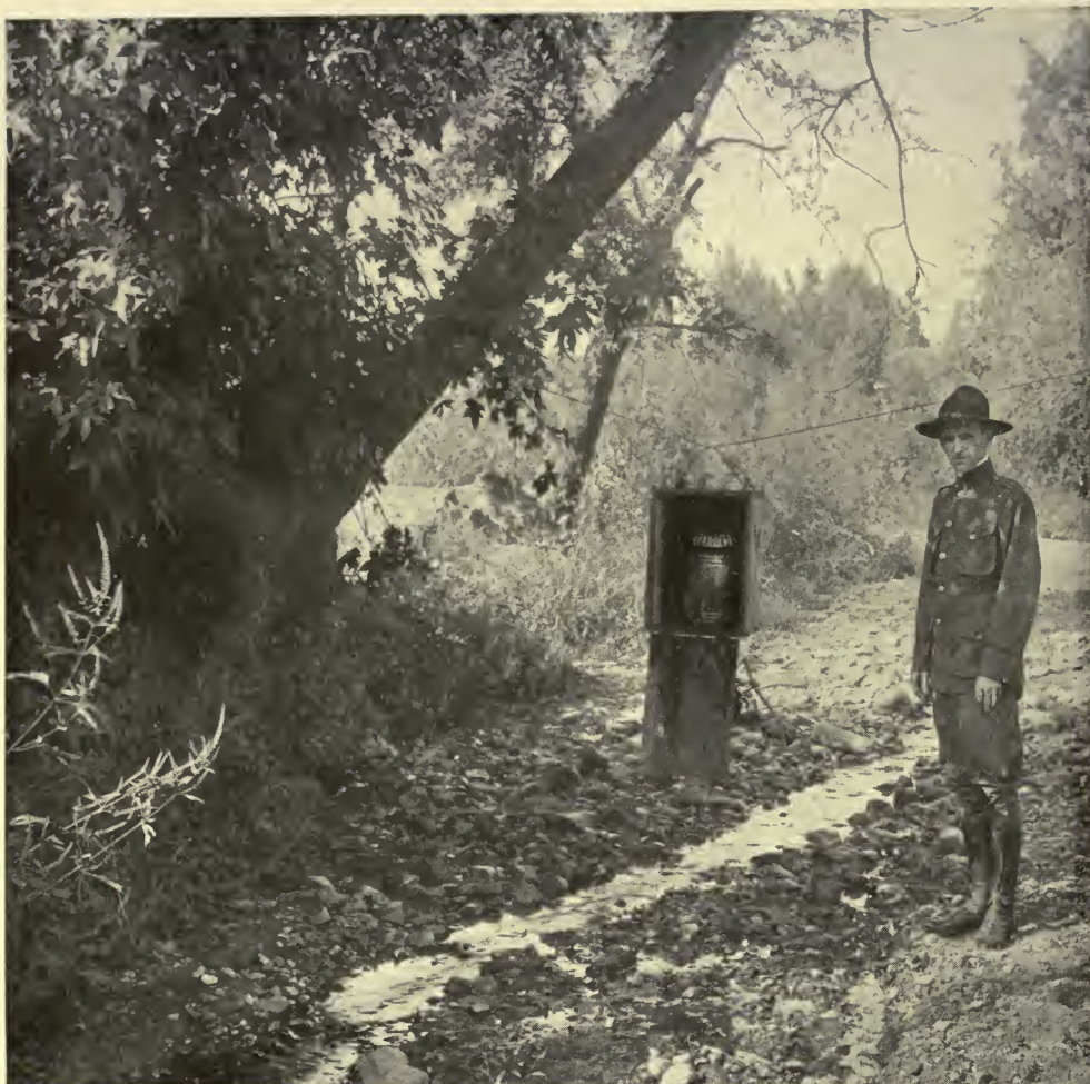
ON STREAMS WHERE THERE IS A PERMANENT FLOW OF WATER, DRIP-CANS ARE INSTALLED TO FURNISH A CONSTANT FILM OF OIL FOR SUCH STREAMS
