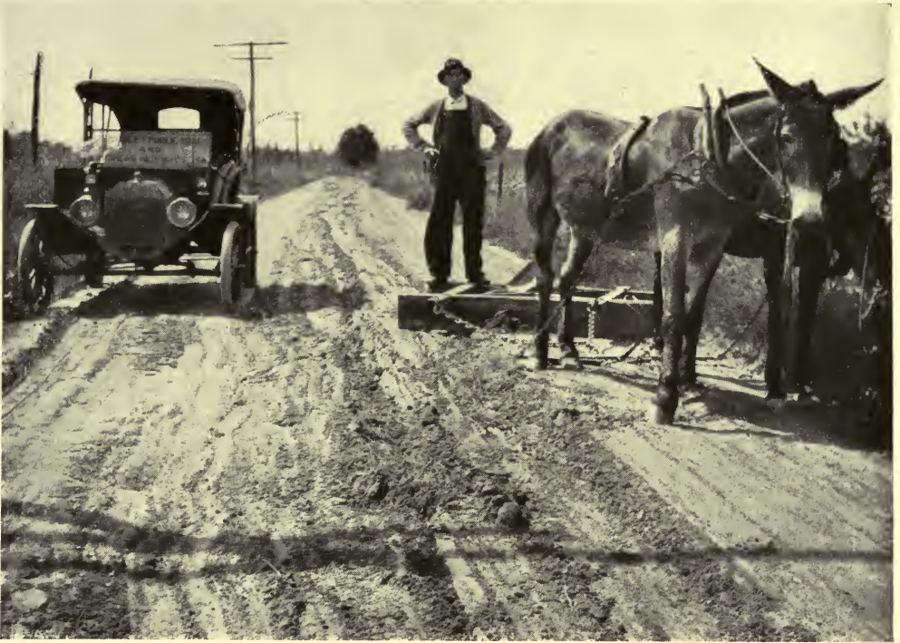
USING A DRAG IN THE IMPROVEMENT OF A ROAD IN NORTH CAROLINA
