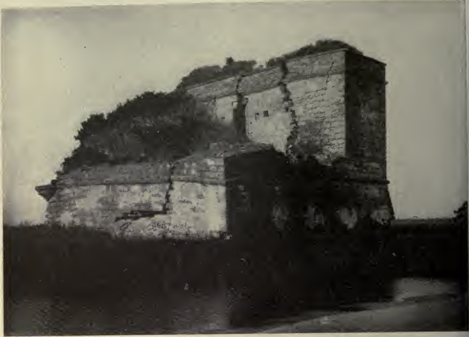
THE OLD SPANISH FORT, MATANZAS INLET, FLORIDA
