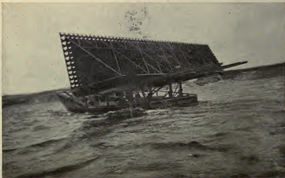
THE CYGNET SAFELY LIFTED ON TO ITS RAFT AND READY TO BE TOWED HOME
