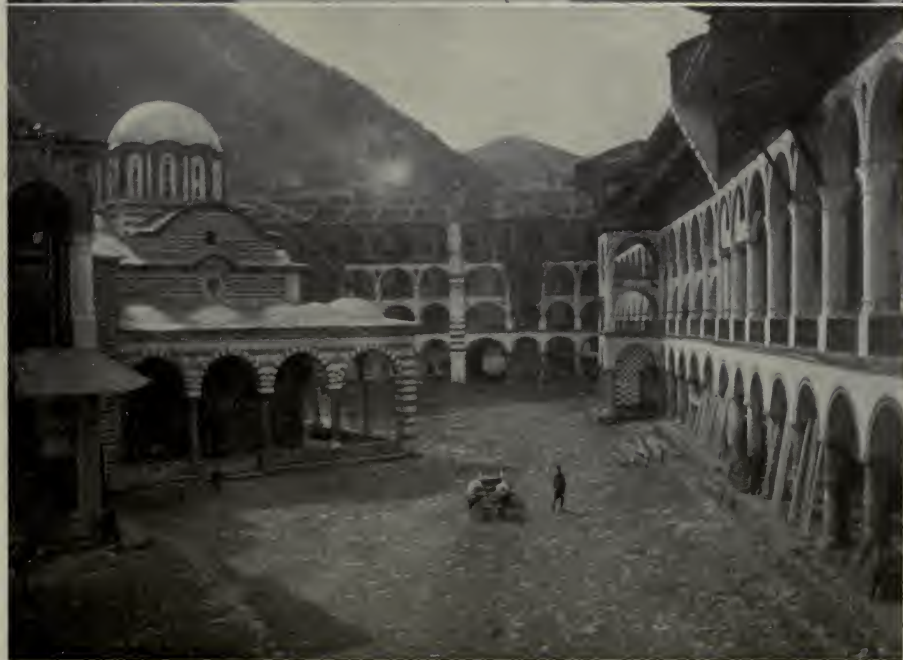
A CORNER OF THE MONASTERY AT RILO
