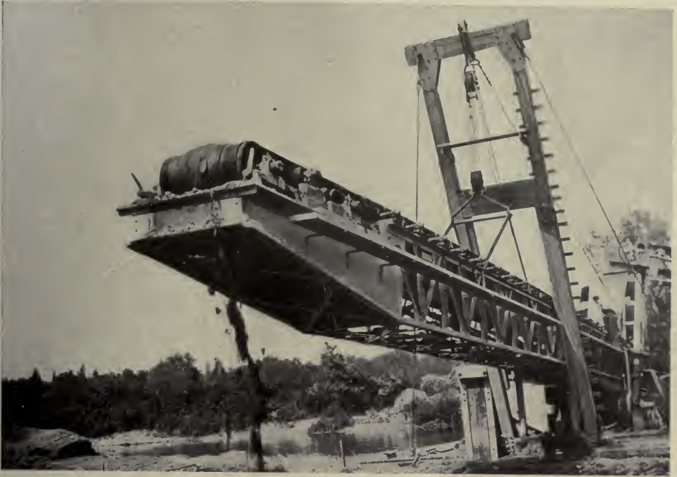
TYPE OF CONVEYOR DREDGE USED IN CHANNEL-DEEPENING
