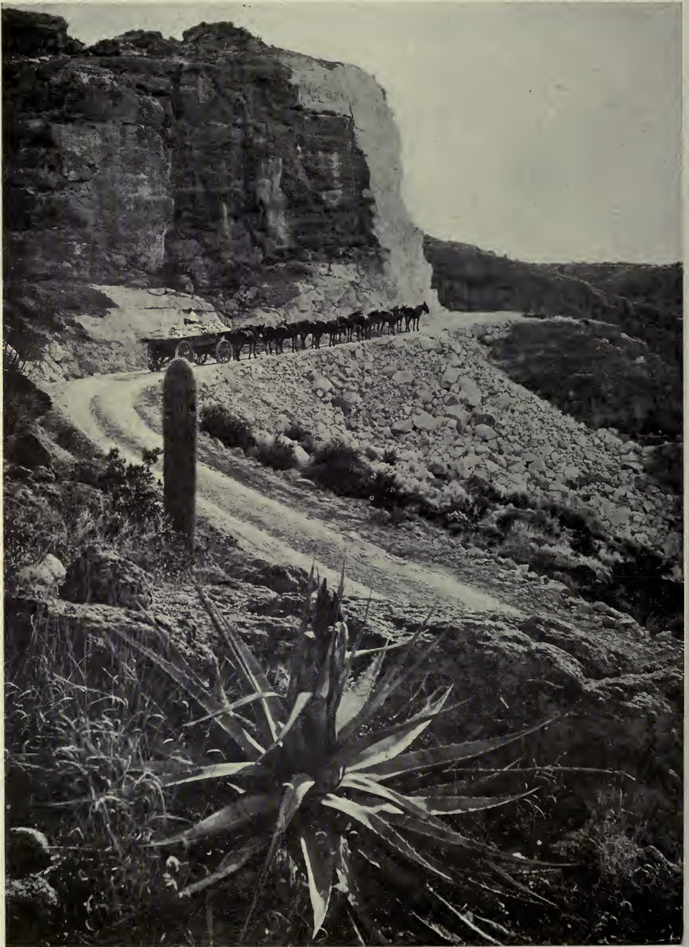
THE TOP OF FISH CREEK HILL, ARIZONA, ON THE MESA AND ROOSEVELT STAGE ROAD, WHICH WAS BUILT BY THE GOVERNMENT: SALT RIVER PROJECT, ARIZONA (SEE PAGE 278)
