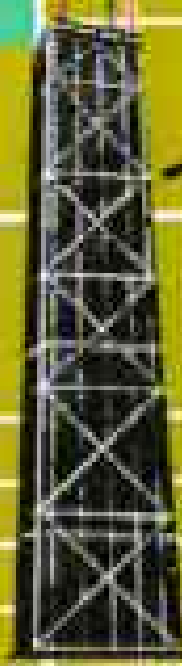
John Hancock Center 1,127 feet
