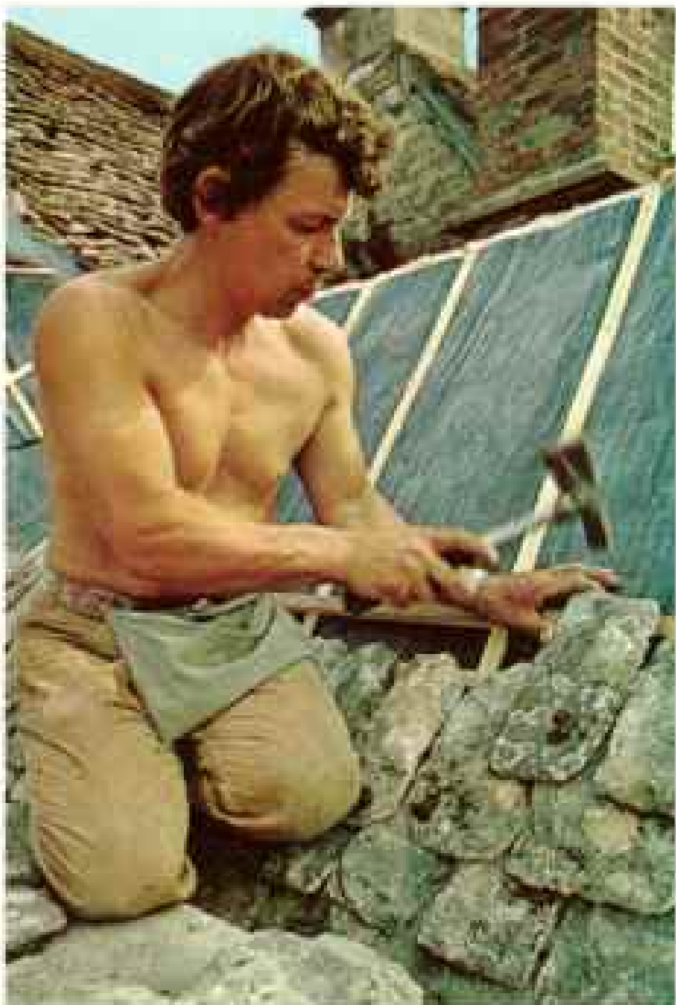
Patching past to present, Roy Agg nails lichen-covered tiles recovered from an old barn to the roof of a Burford shop.
