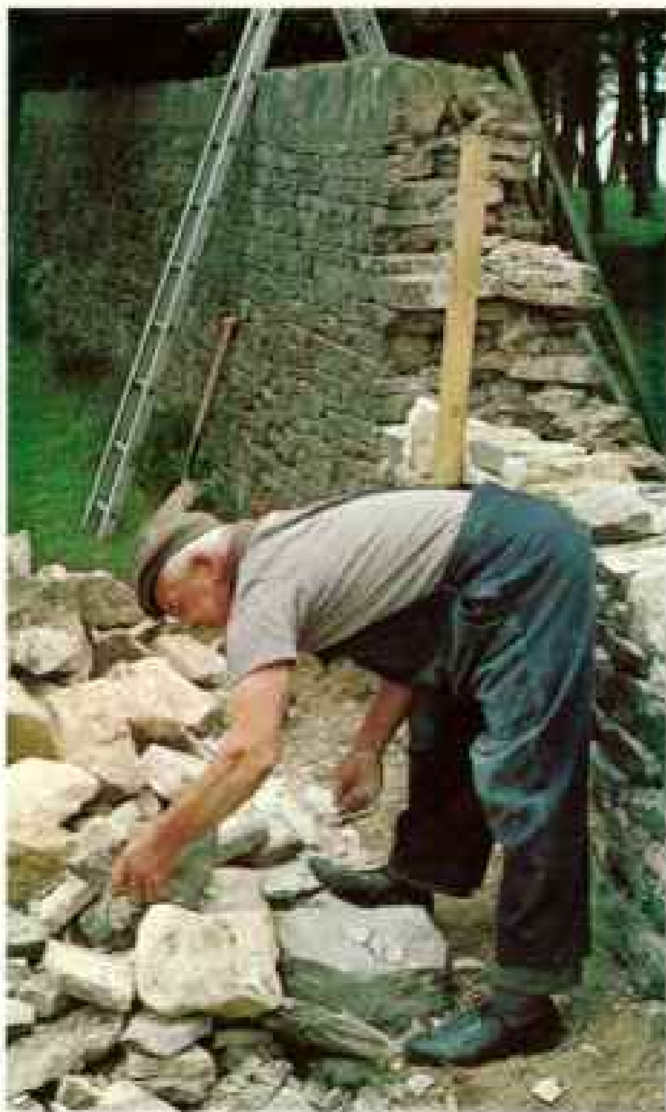
"She's loike a jigsaw puzzle," declares mason William Pulham (above), as he repairs a traditional dry wall of intricate pattern.
