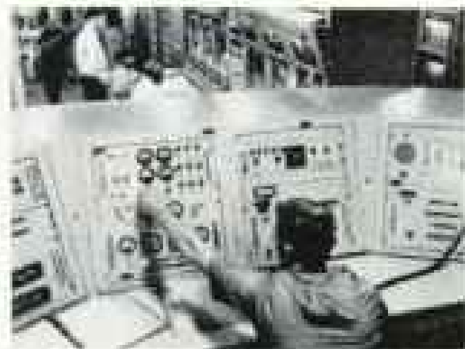
Control Room For 20-foot diameter Starboard Antenna
