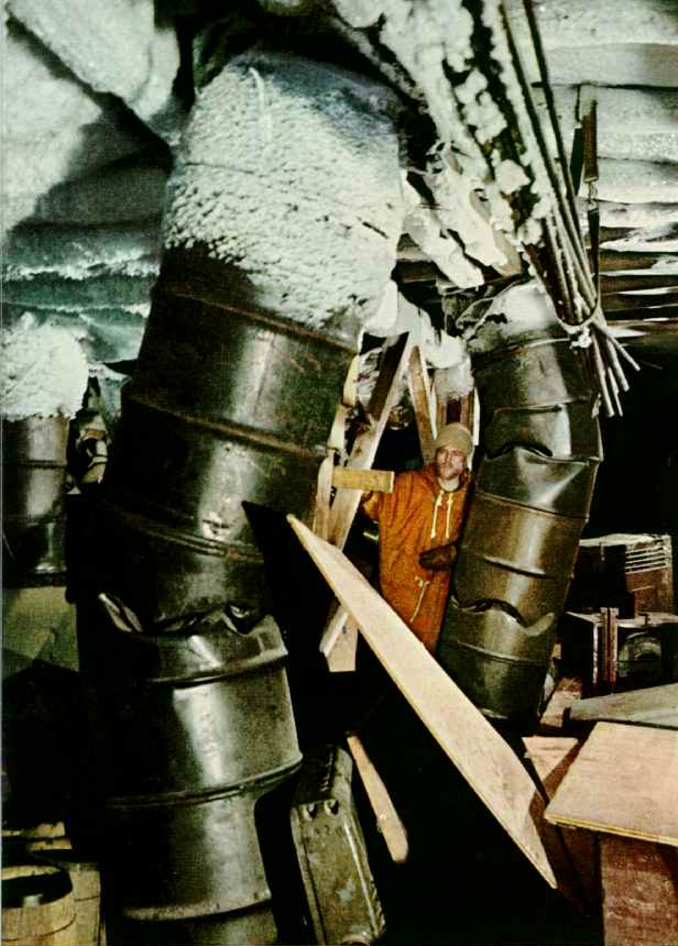
Oil-drum pillars crumple at old Byrd Station. Roof sags under tons of crushing snow
