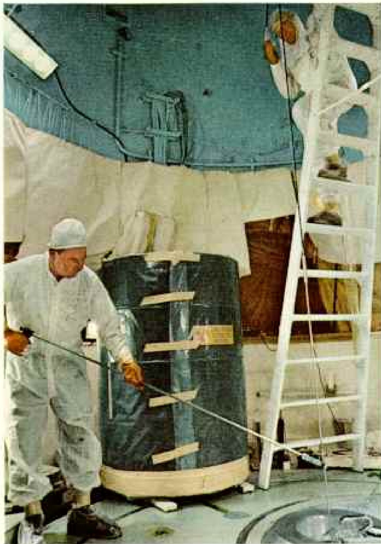
Keeping their distance, technicians lower a neutron-emitting starter into the core. To lessen exposure, they practiced until they could do the job in ten seconds.
