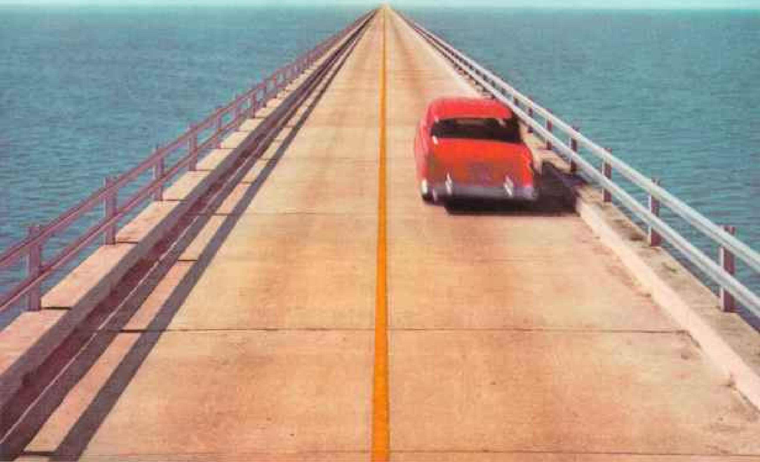
Seven-Mile Bridge on Florida's Key West Causeway—one of America's longest open-water bridge crossings.
