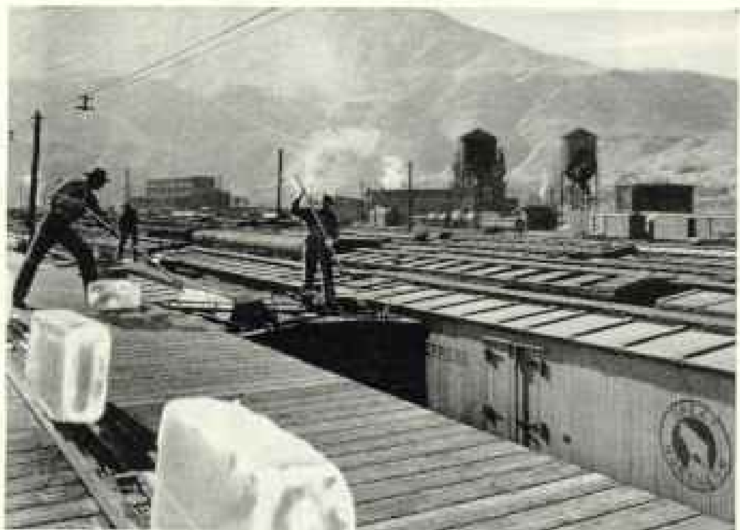
Pre-cooling of refrigerator cars before loading is important. This requires thousands of tons of ice each shipping season. Heaters protect apples from midwinter temperatures.
