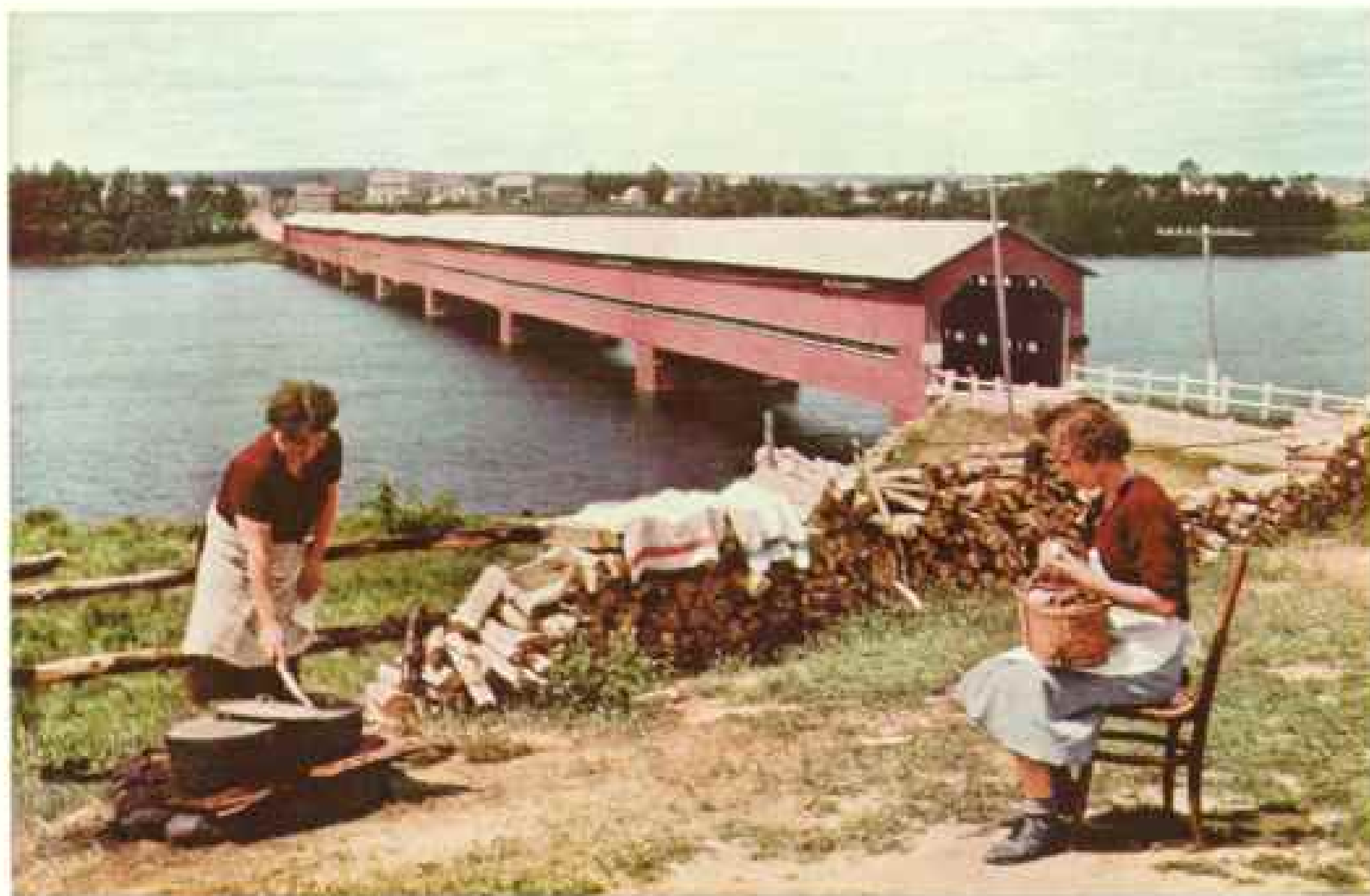
COVERED BRIDGES WHICH SAVE SNOW SHOVELING ARE LONG LIVED
