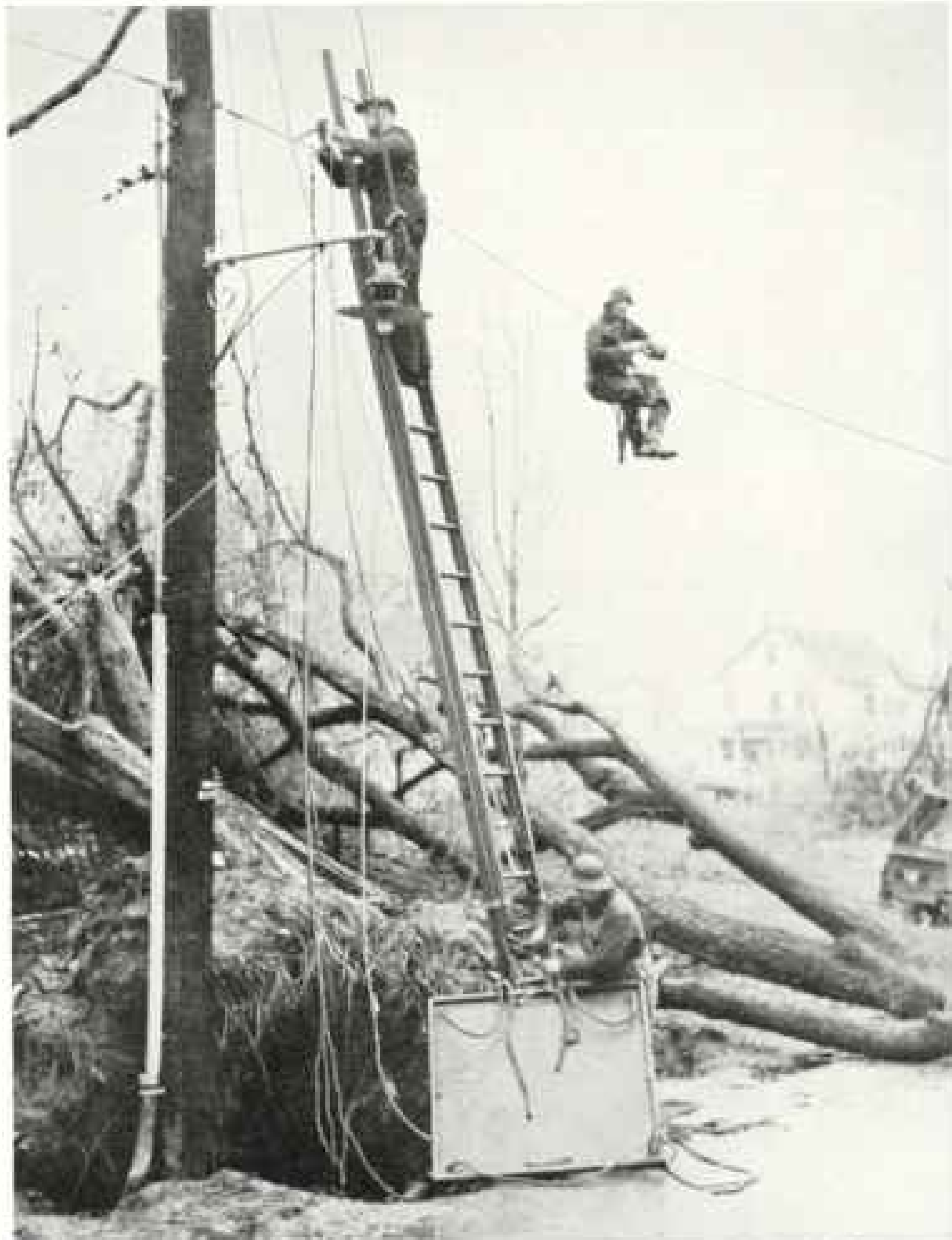
Photograph courtesy New England Telephone and Telegraph Company
