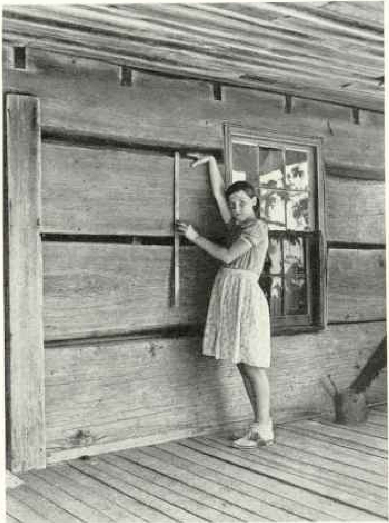
MASSIVE TIMBERS WENT INTO CABIN WALLS.
