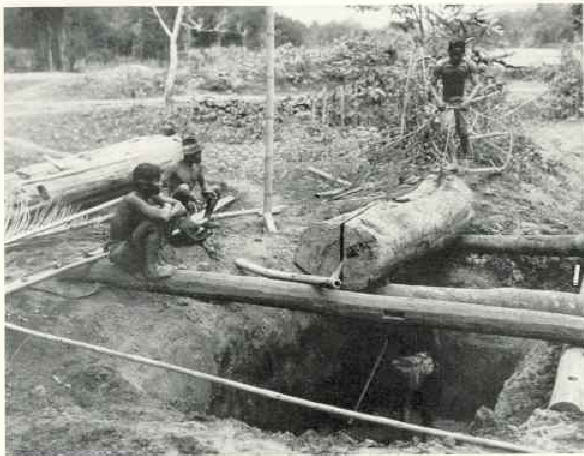
A PIT SOLVES THE PROBLEM OF SAWING HEAVY TEAK LOGS
