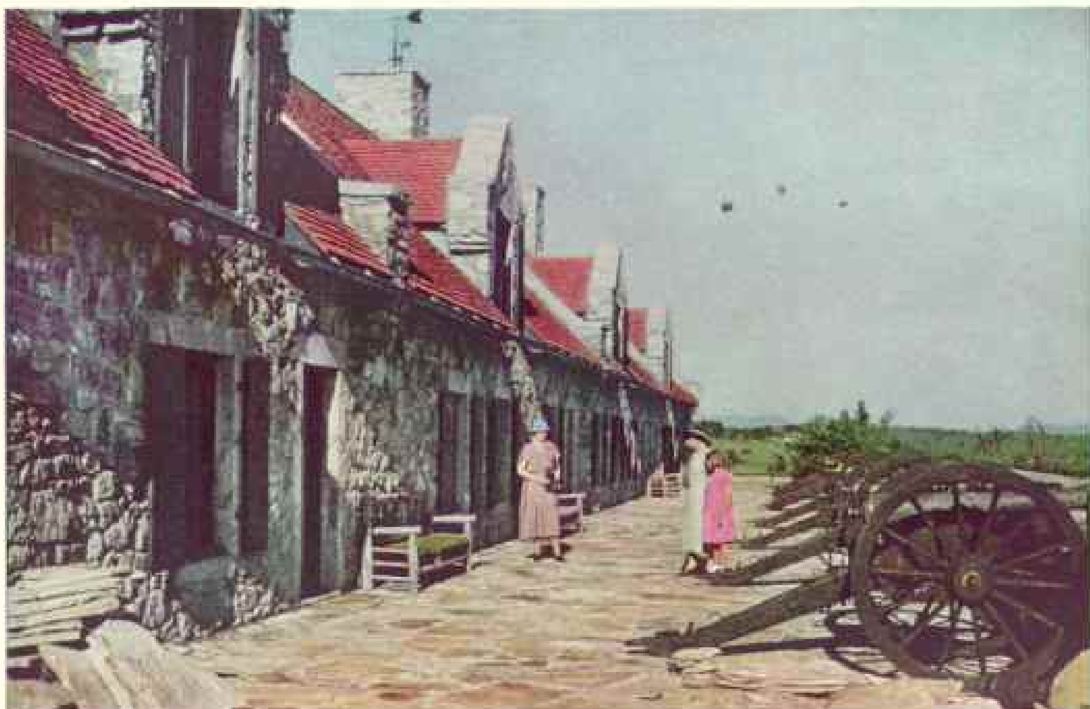
THE RESTORED SOUTH PLATFORM AT FORT TICONDEROGA
