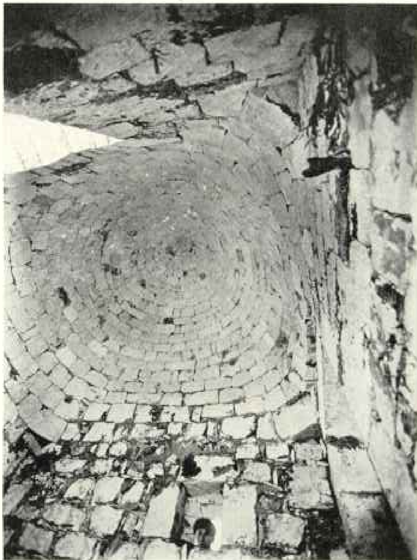
TRULLI ARE LAID UP FROM WITHIN LIKE CISTERNS
