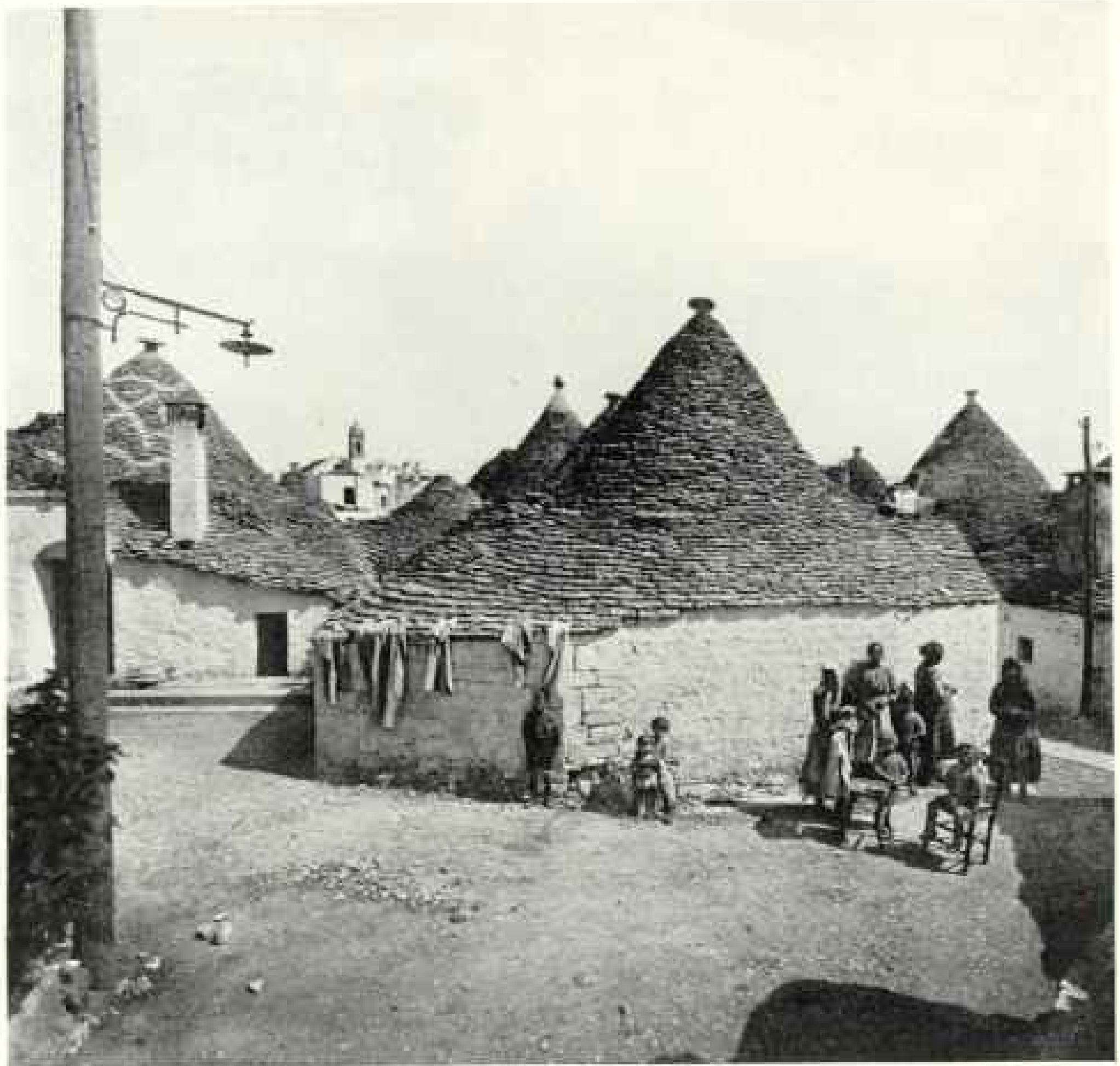
PROGRESS REACHES THIS TRULLI VILLAGE IN THE FORM OF ELECTRIC STREET LIGHTING
