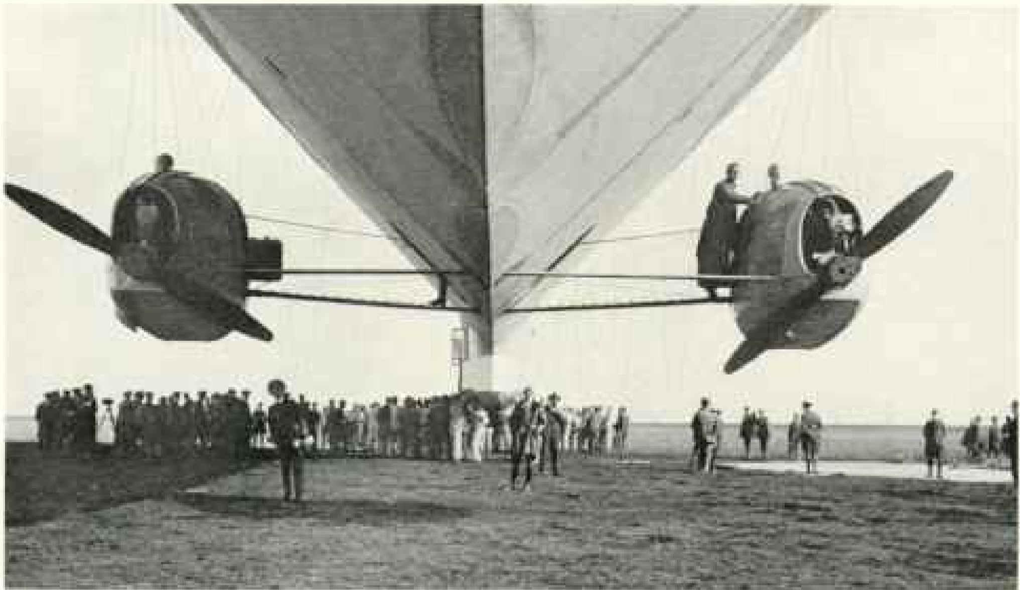
THE LATERAL ENGINE BOATS OF THE "NORGE," SHOWING THE CATWALK BETWEEN KEEL AND ENGINE BOAT
