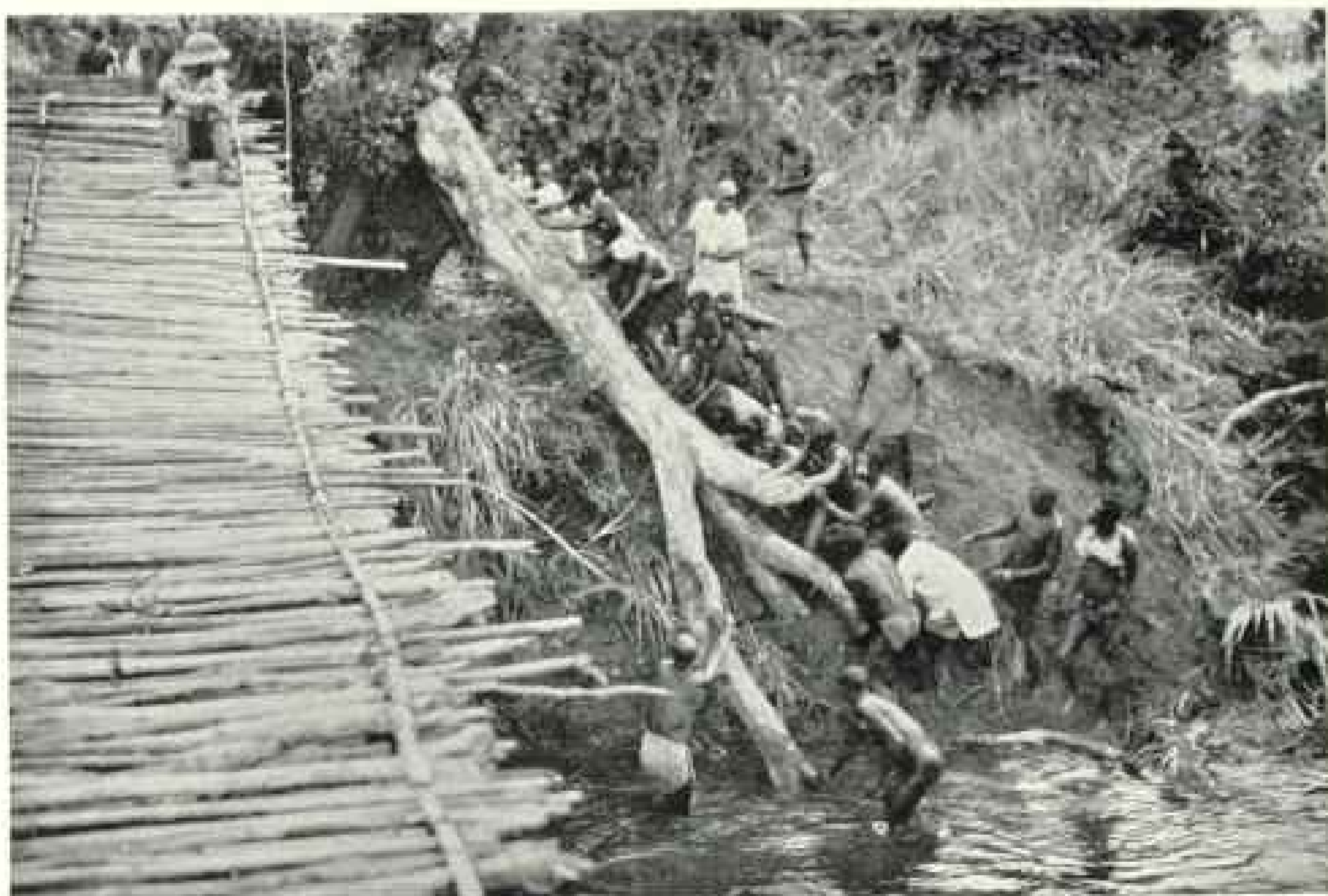
STRENGTHENING A NATIVE BRIDGE FOR THE CATERPILLAR CARS
