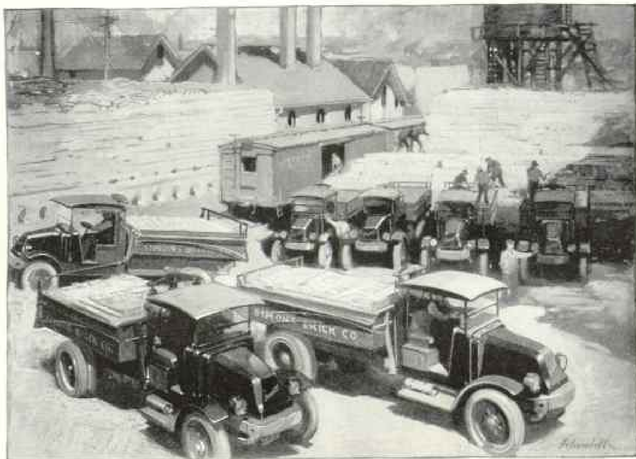
Part of a Fleet of Sixteen Internationals Serving the Simon's Brick Co. of Los Angeles
