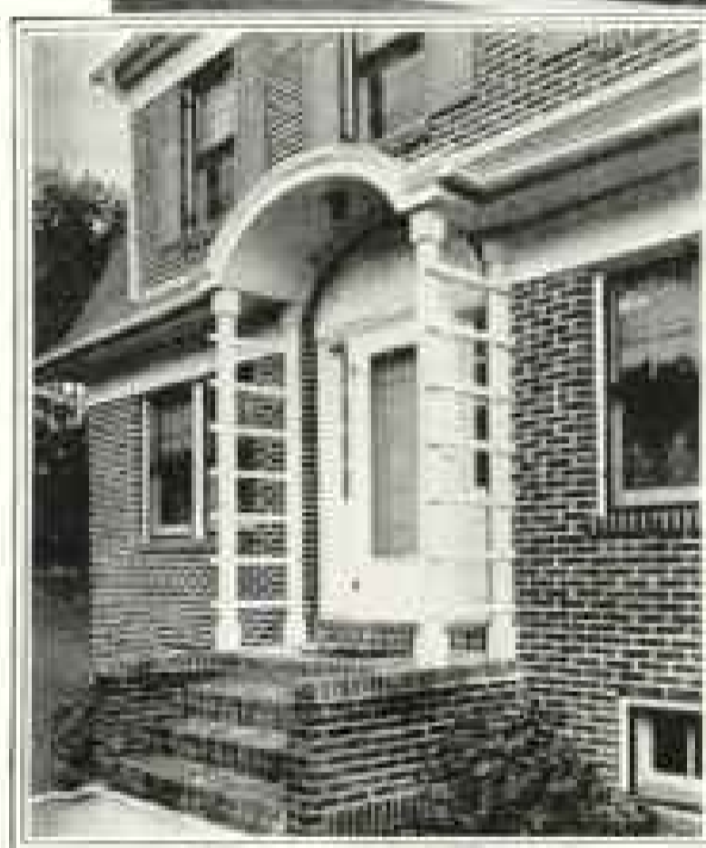
A. F. B. A. HOUSE No. 638 at Park Ridge, Illinois
