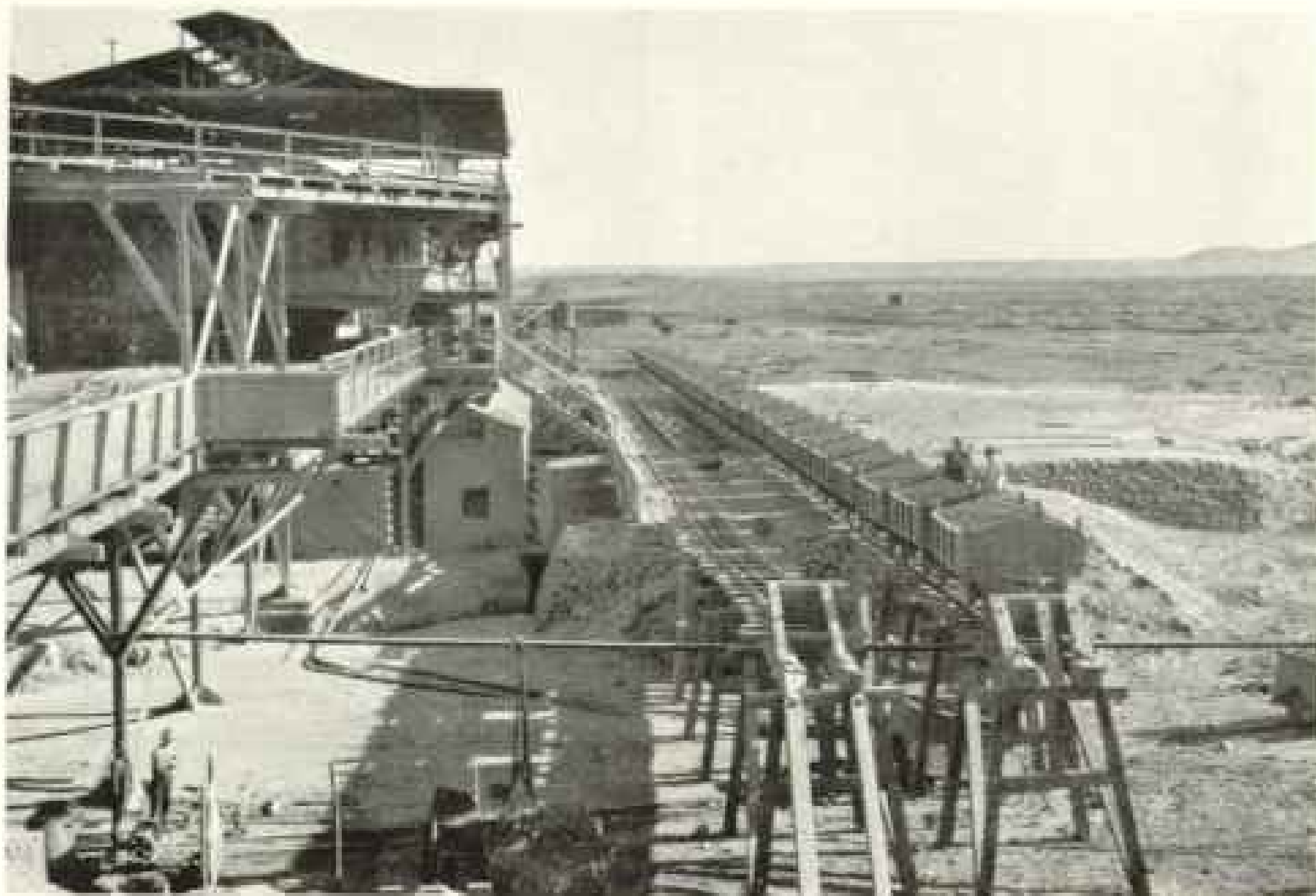
A NITRATE PLANT OF NORTHERN CHILE
