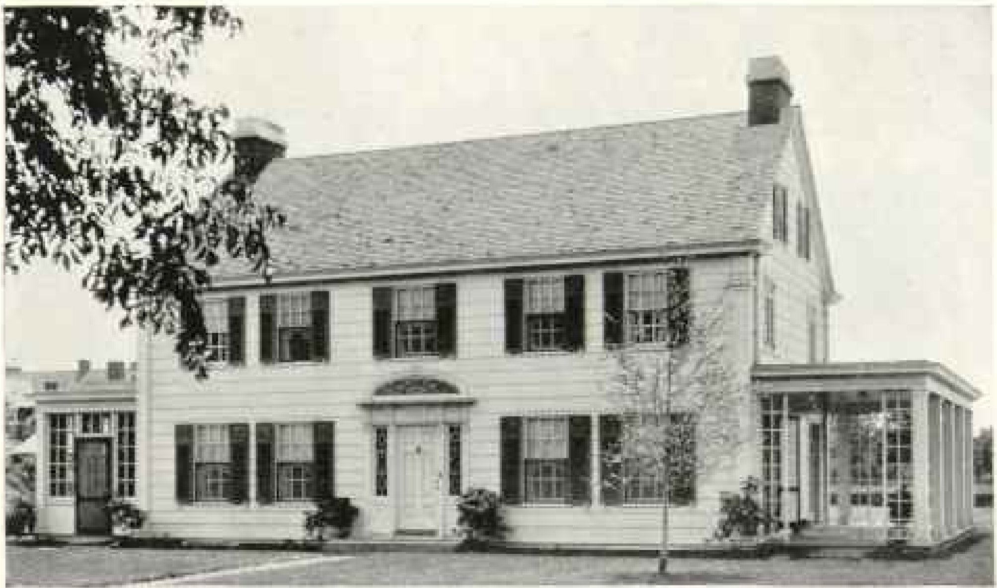
House of F. P. Clarke, Esq., Garden City, N. Y. Aymar Embury II, Architect, New York City.
