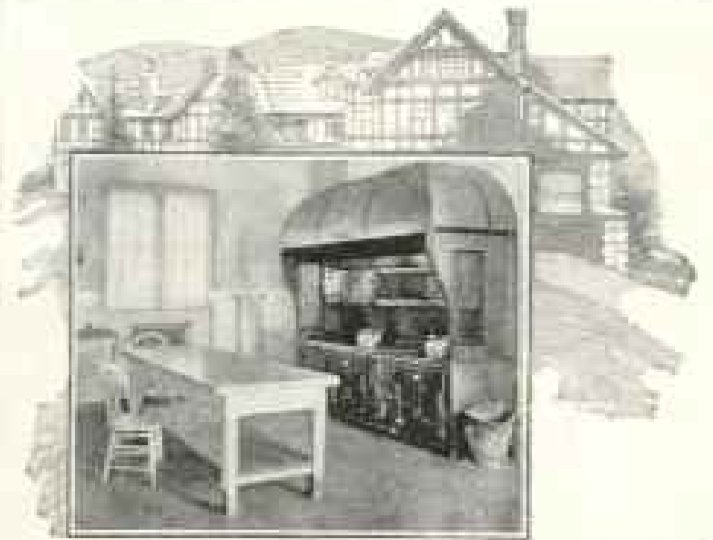
Electric and Fuel Ranges and Dining Table in the Home of A. L. Janssen, Greenwich, Connecticut. C. P. H. Gilbert, Architect
