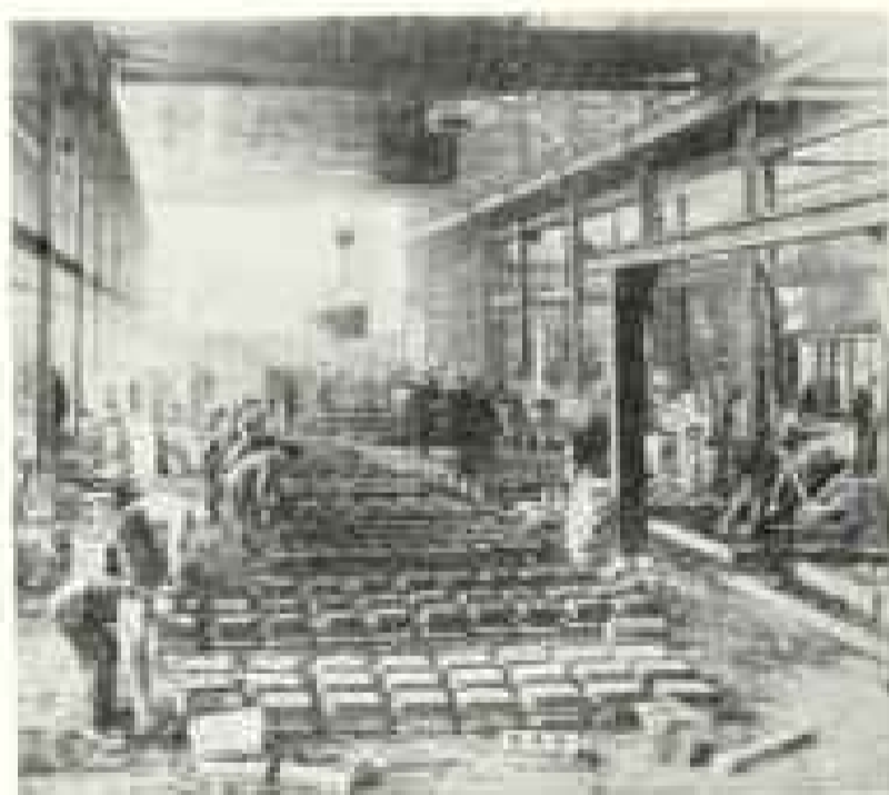
Cool air thru the side ventilators replaces fumes and gases which rise steadily to the monitor exits of this foundry
