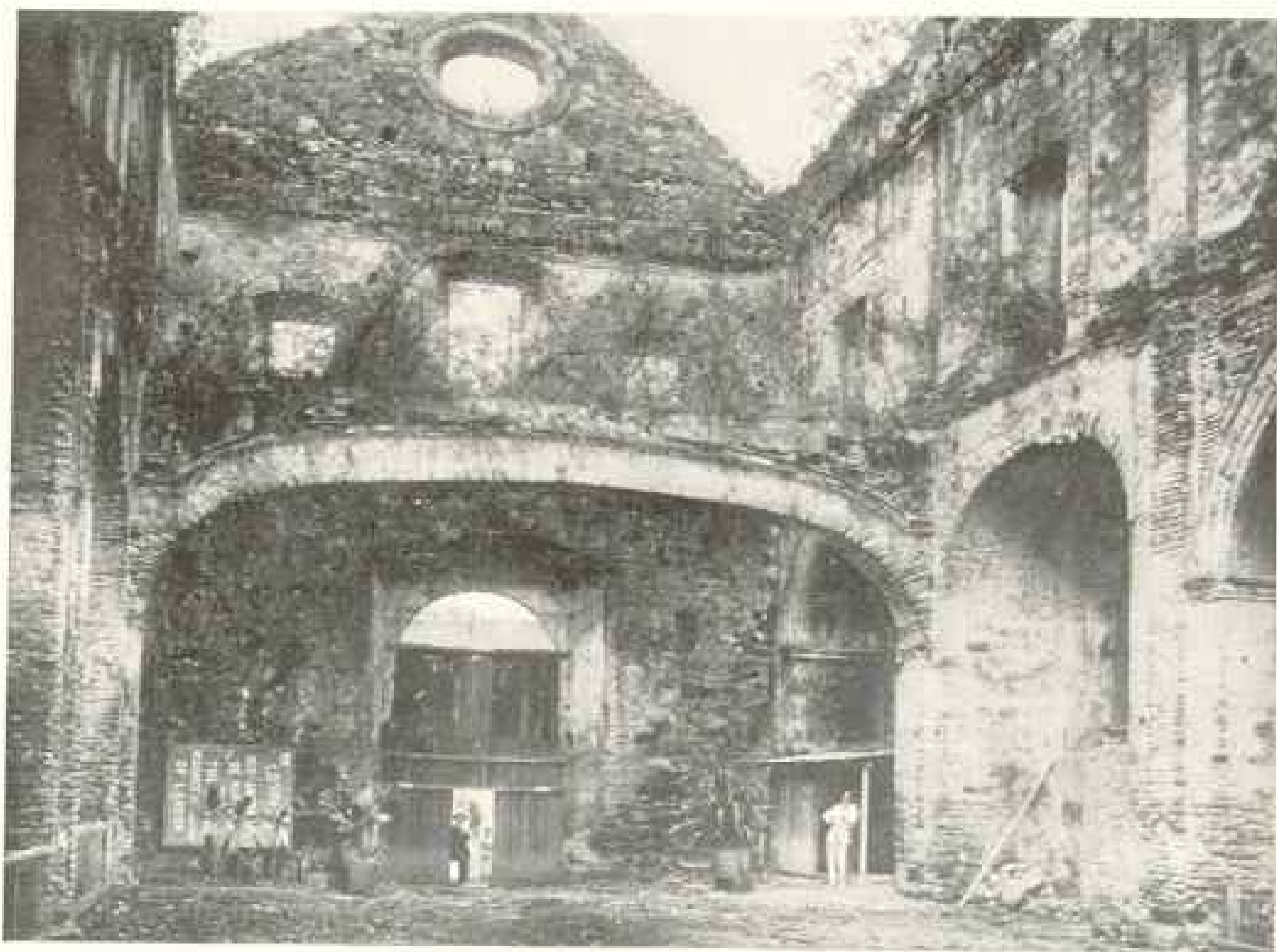
THE FLAT ARCH AT PANAMA
