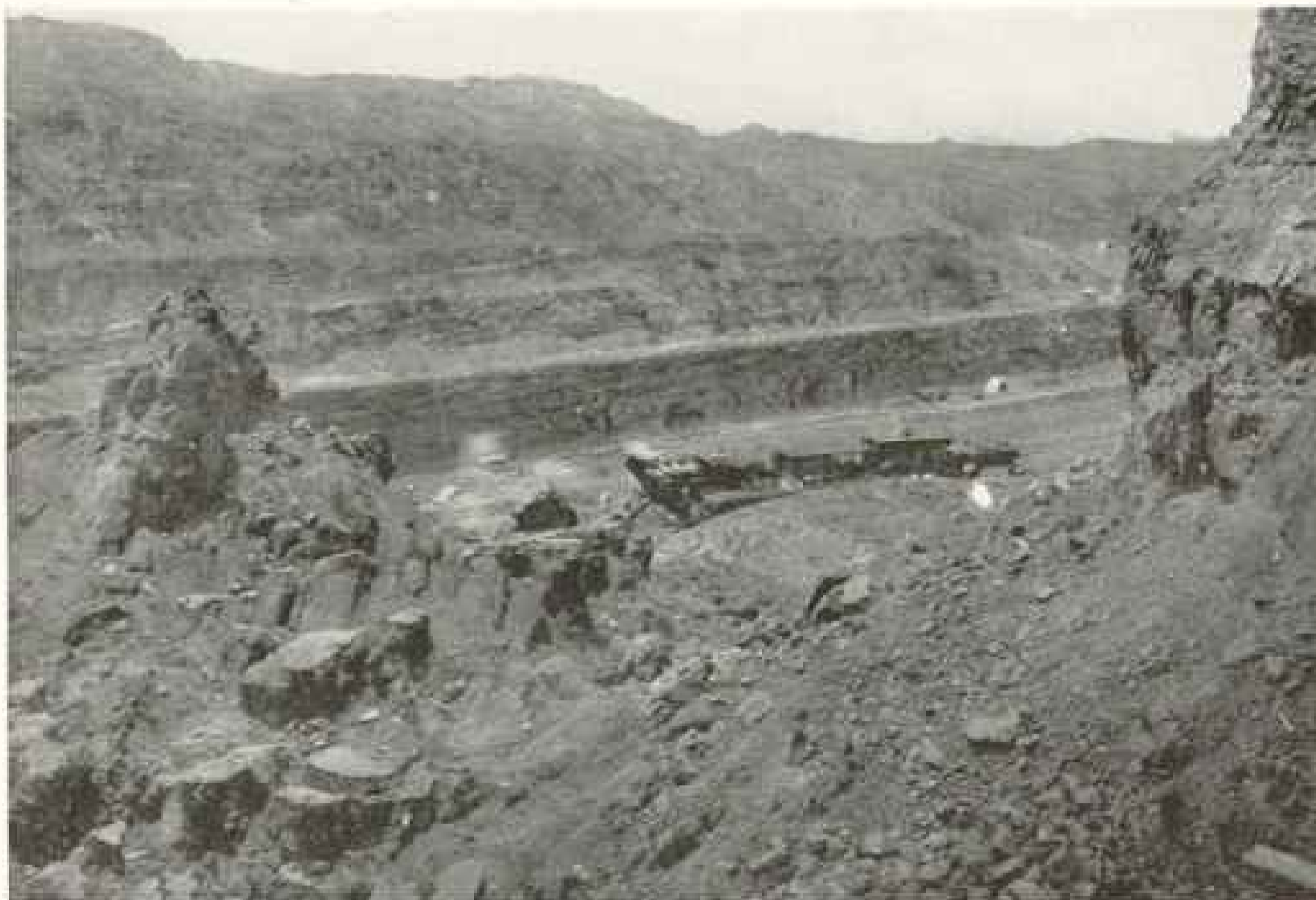
LOOKING INTO THE CULERRA CUT FROM THE TOP OF A SLIDE, SHOWING THE BROKEN BANK
