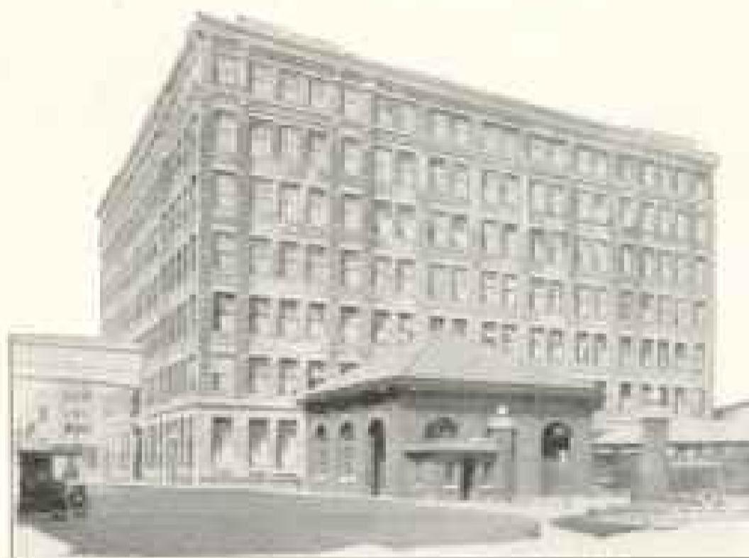
New building of the G-E Research Laboratories at Schenectady, headquarters for the scientific effort known as "Mazda" Service. This Service synthesizes constant experimentation and world-wide investigation, so that the mark "Mazda" on an electric lamp shall always signify the latest achievements in metal filament lighting by the ablest lamp experts in the world.
