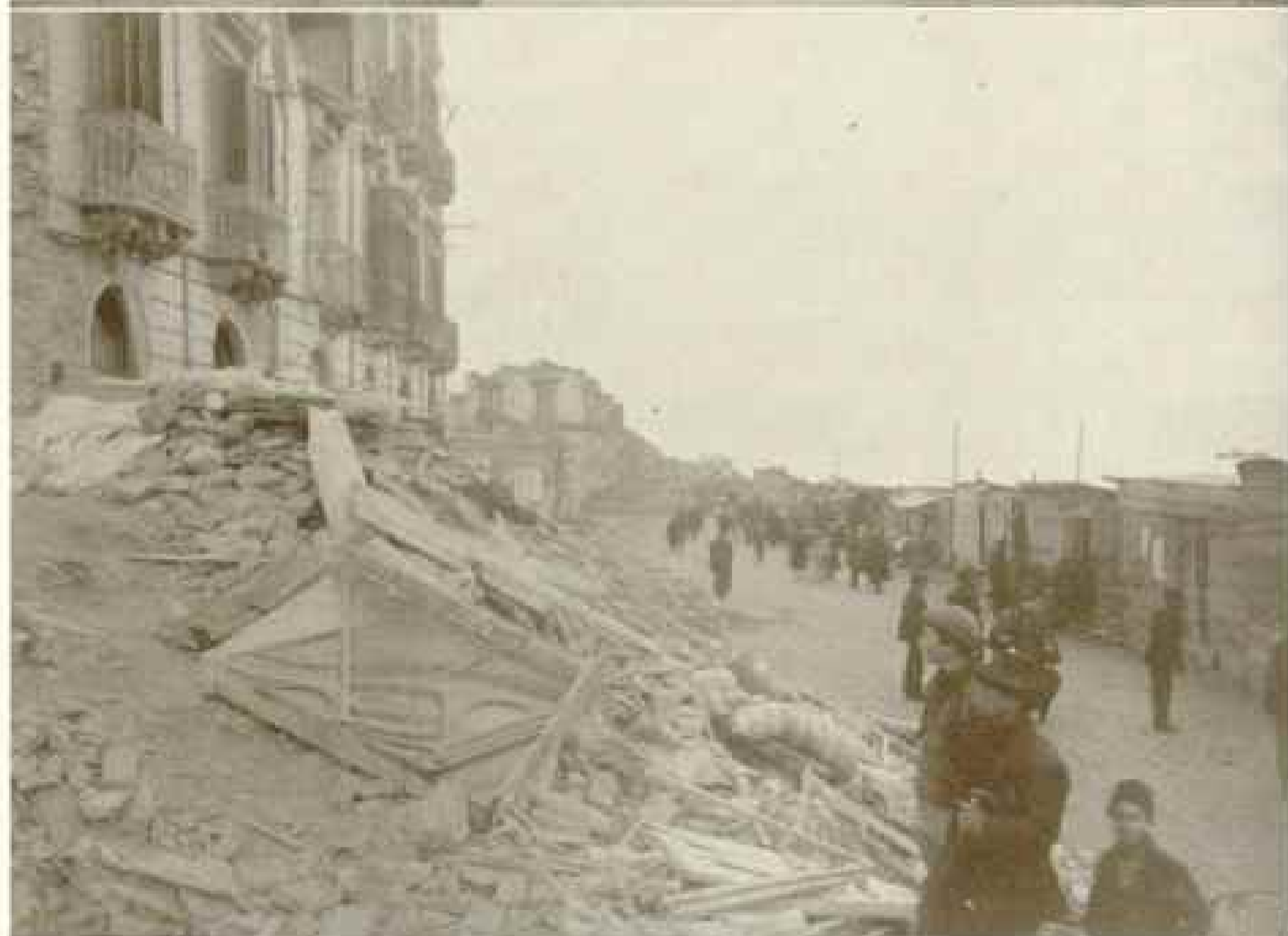
CORSO VITTORIO EMMANUELE LOOKING NORTH ALONG WATER FRONT IN MESSINA Showing the local displacement of the quay, even below water level, and the destruction of the famous Palazzata, "the pride of Messina"
