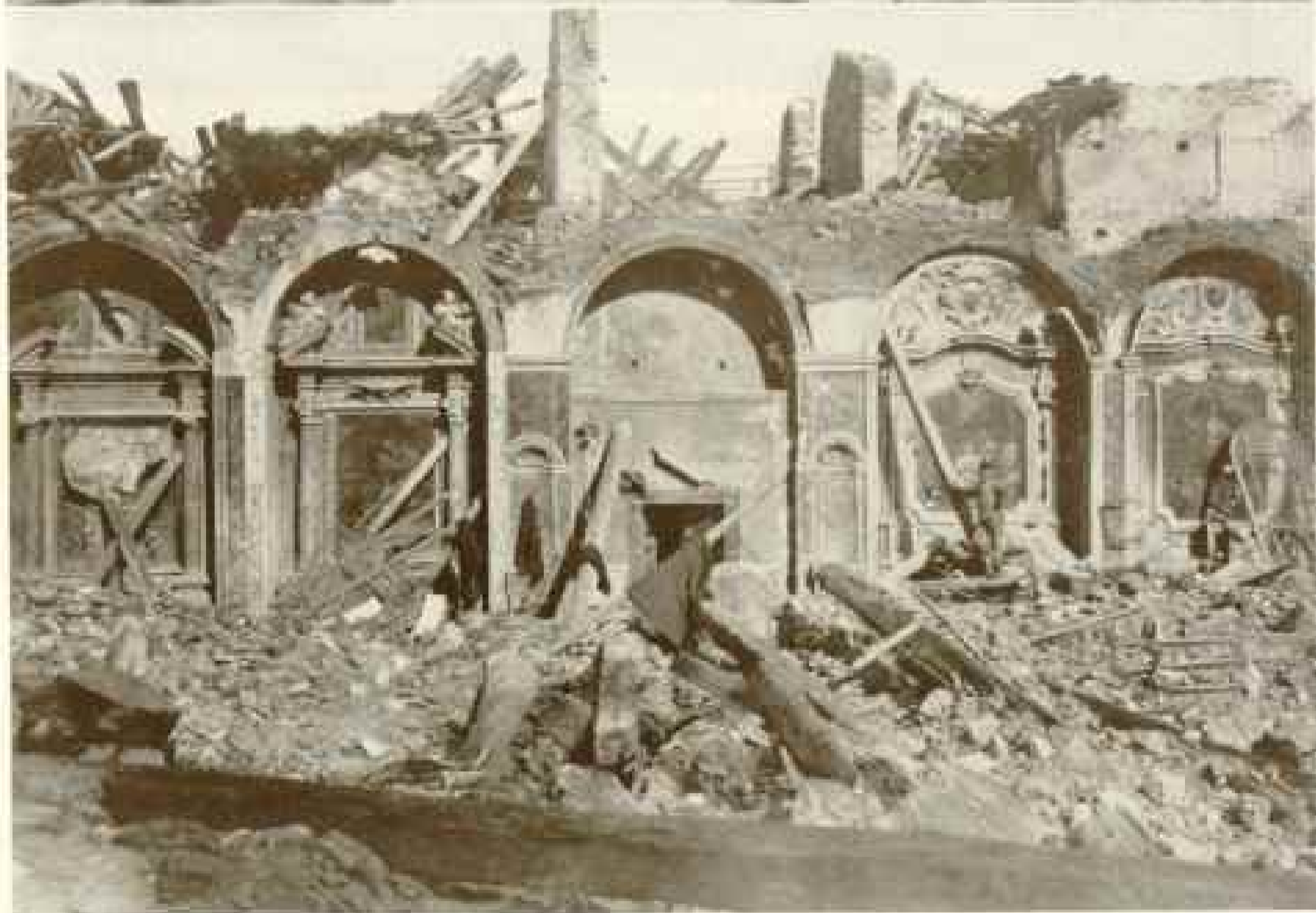
INTERIOR OF DUOMO AT MESSINA SHOWING ROW OF SAINTS, SOME HAVING BEEN THROWN OUT OF THEIR BERTHS BY THE SHOCK
