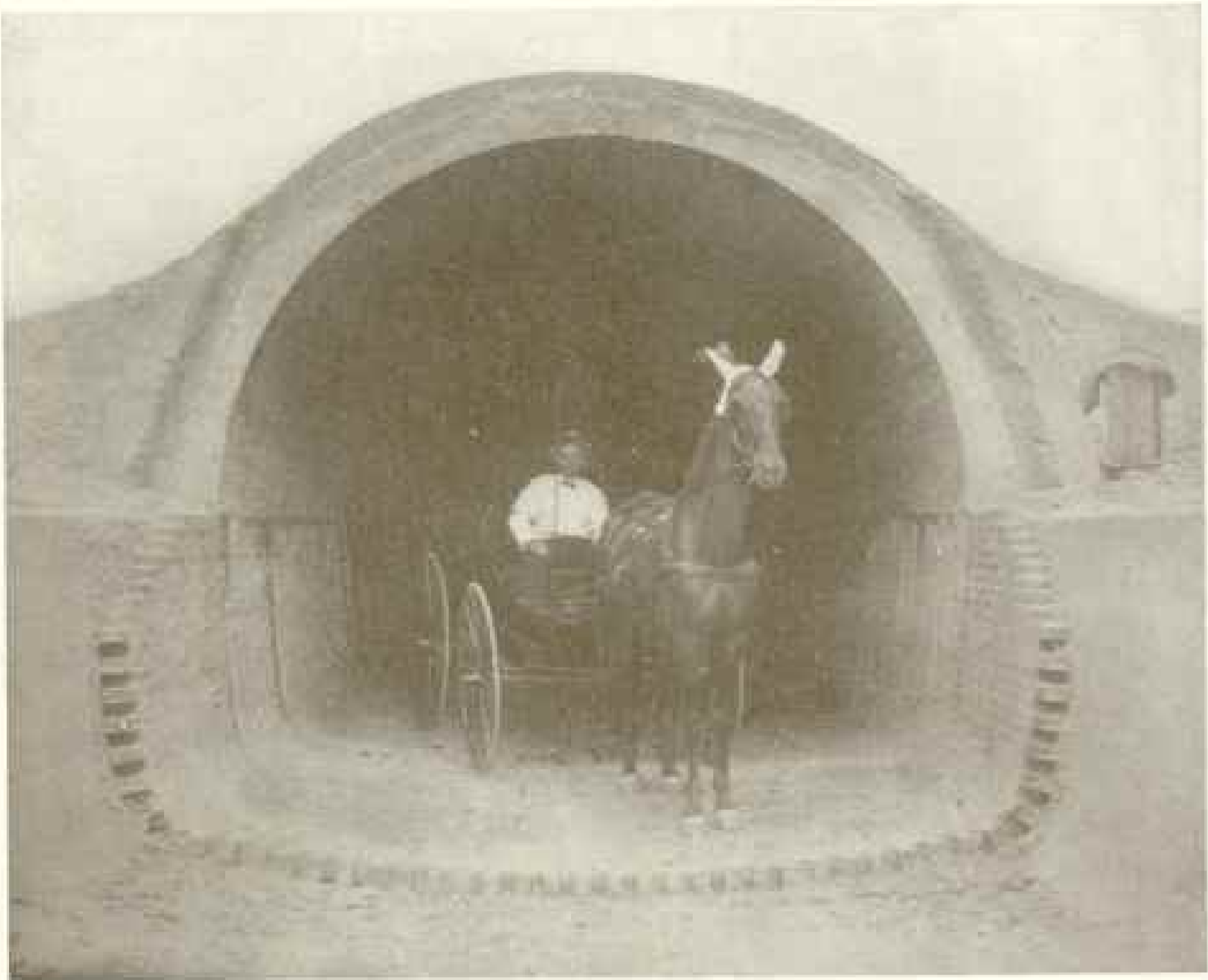
A COMPLETED SECTION OF THE OUTFALL SEWER
