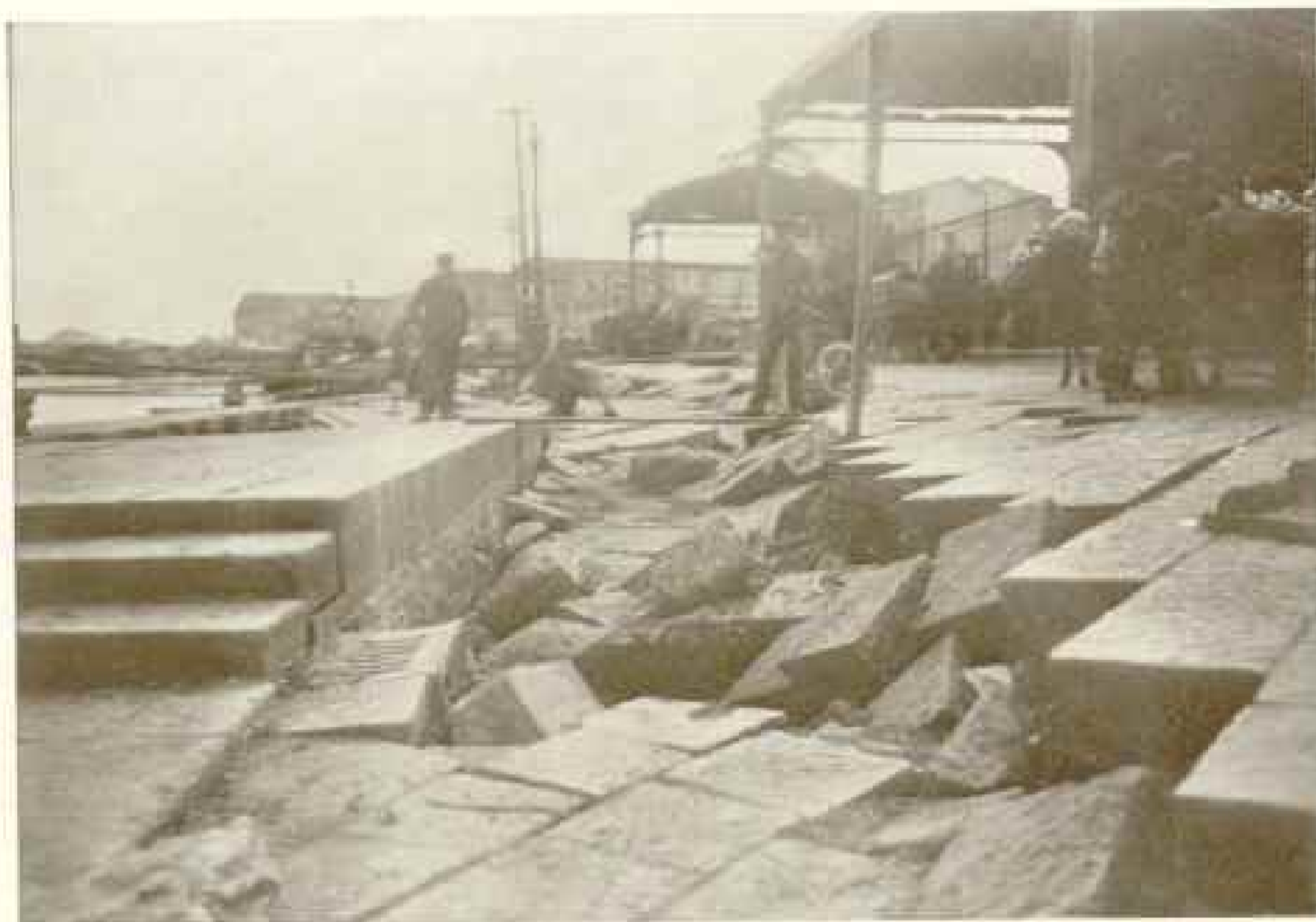
VIEW ALONG QUAY IN MESSINA SHOWING A DISPLACEMENT CAUSED BY LOCAL LAND-SLIPPING
