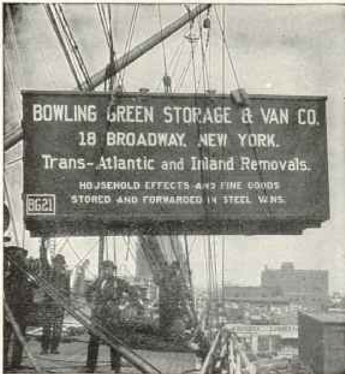
HOISTING LIFT-VAN ON BOARD STEAMSHIP
