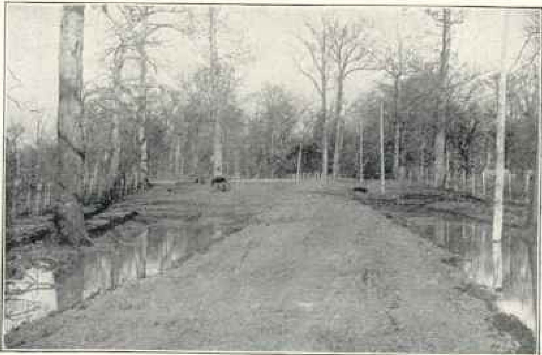
Partial View of Finished Road
