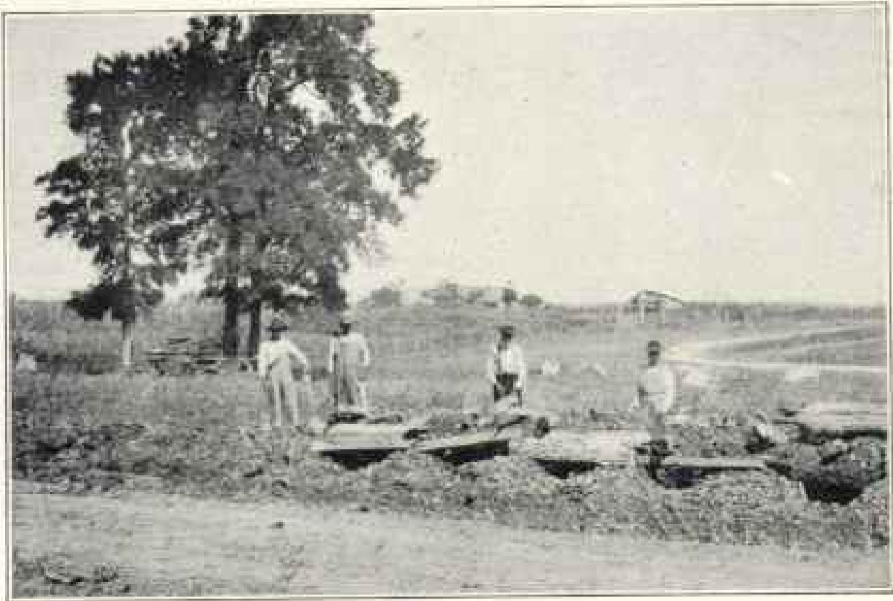
First and Second Courses of Wood Covered with Lump Clay
