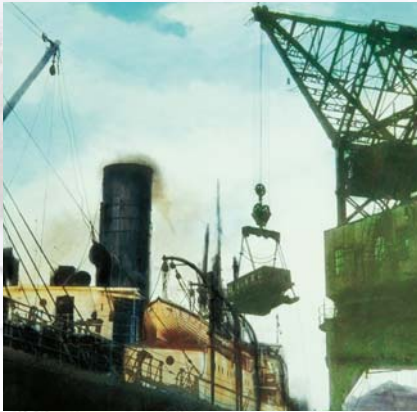
Loading coal at the docks
