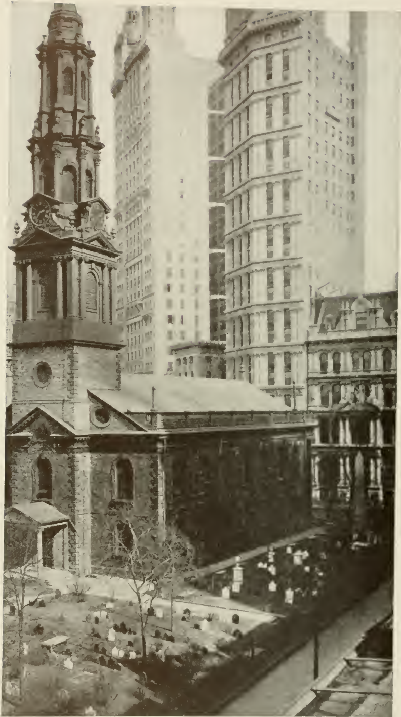
ST. PAUL'S CHAPEL. ENGLISH COLONIAL. McBEAN. 1764—66. STEEPLE. 1794 ST. PAUL BUILDING (MIDDLE RIGHT) POST. C. 1898 PARK ROW BUILDING (MIDDLE LEFT) FUNCTIONAL STYLE. ROBERTSON. 1896—98 New York City
