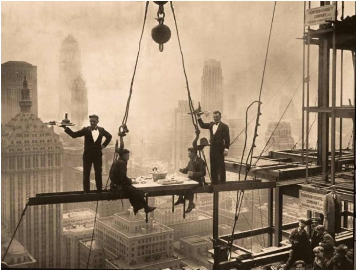
Above: Two waiters serve lunch to steel workers at the Waldorf Astoria Hotel while it was under construction in 1930 (Photo: Keystone/Getty Images)
