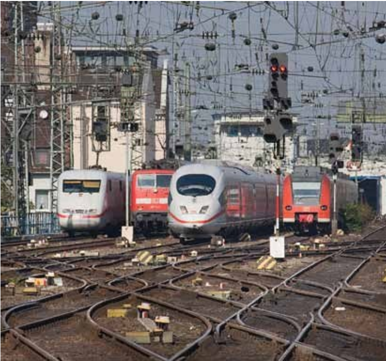
Figure 12.1 Cologne train station, view of the tracks leading into the station, and the complex overhead wiring.
