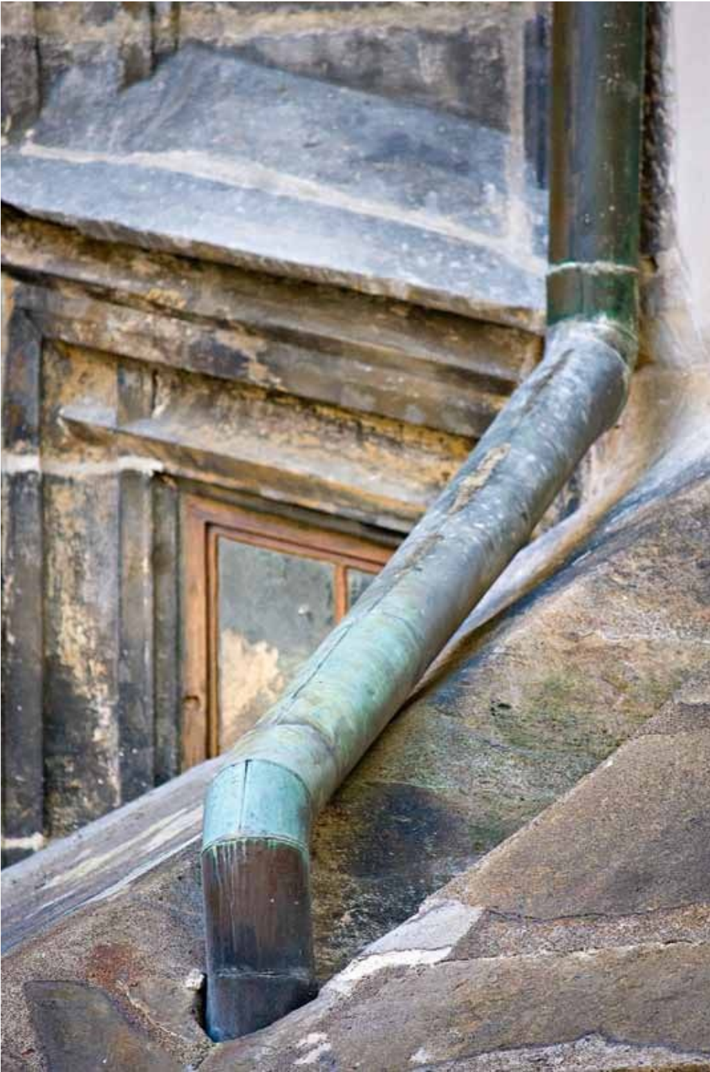
Figure 12.13 Drainpipe – Prague Castle.
