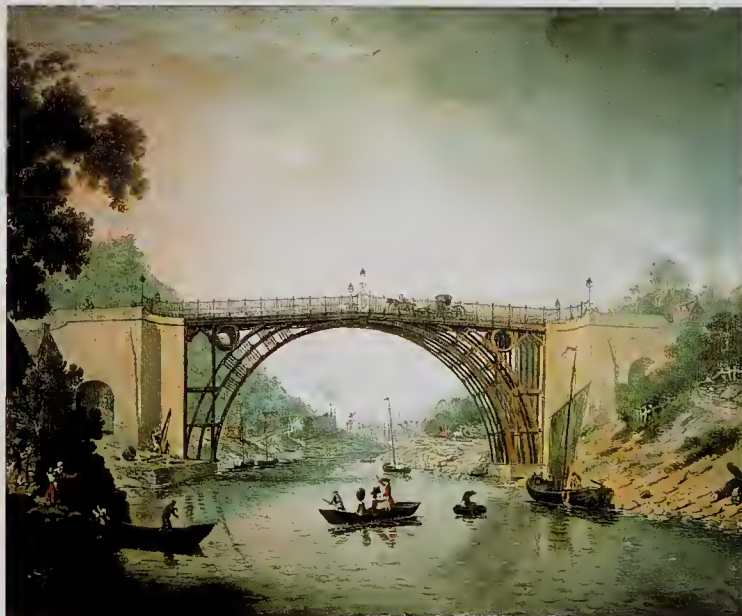
Above A cast iron bridge, built in 1779, spans the river Severn, Britain.
