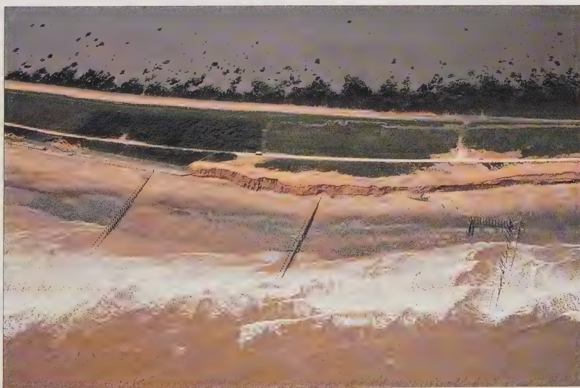
◄ To prevent coastal erosion, groynes are often built that are designed to prevent the loss of sediments through the action of longshore drift. The construction of groynes results in sediment build-up on the up-current side and enhanced erosion on the down-current side.
