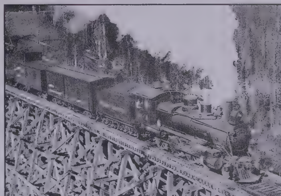
A Canadian Northern train accelerates across a newly built wooden trestle bridge.
