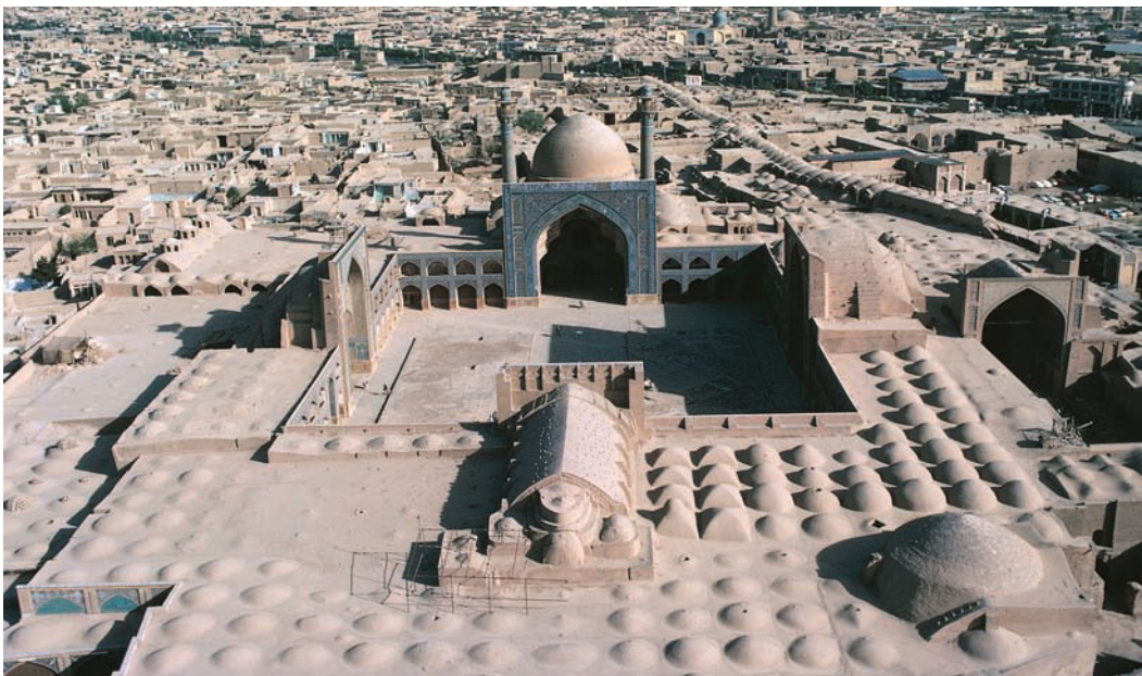
5-10 Aerial view (looking southwest) of the Great Mosque, Isfahan, Iran, 11th to 17th centuries.
