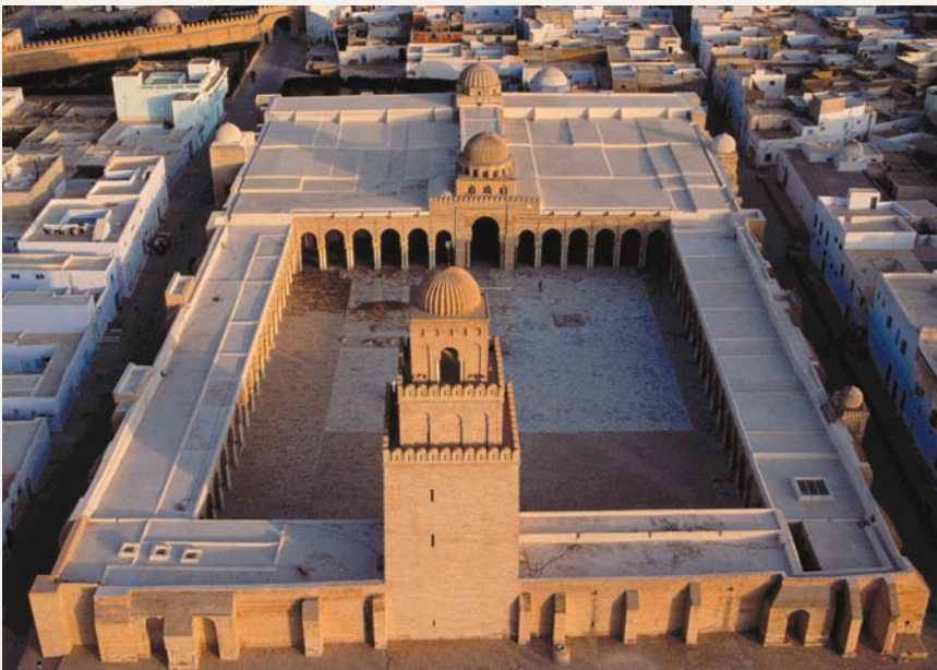
5-4 Aerial view (above) and plan (right) of the Great Mosque, Kairouan, Tunisia, ca. 836–875.
