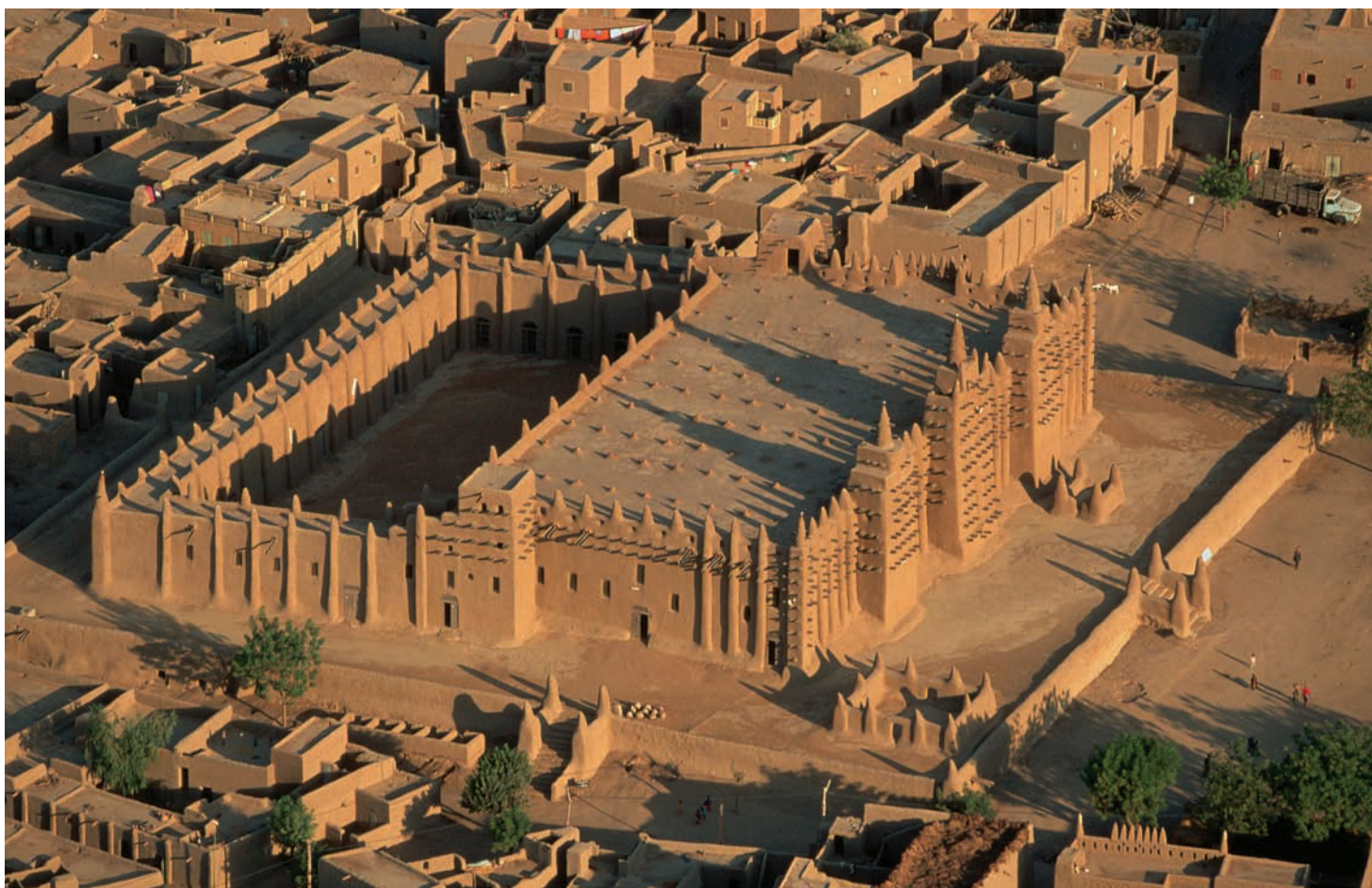
20-5 Aerial view (looking northwest) of the Great Mosque, Djenne, Mali, begun 13th century, rebuilt 1906–1907.
