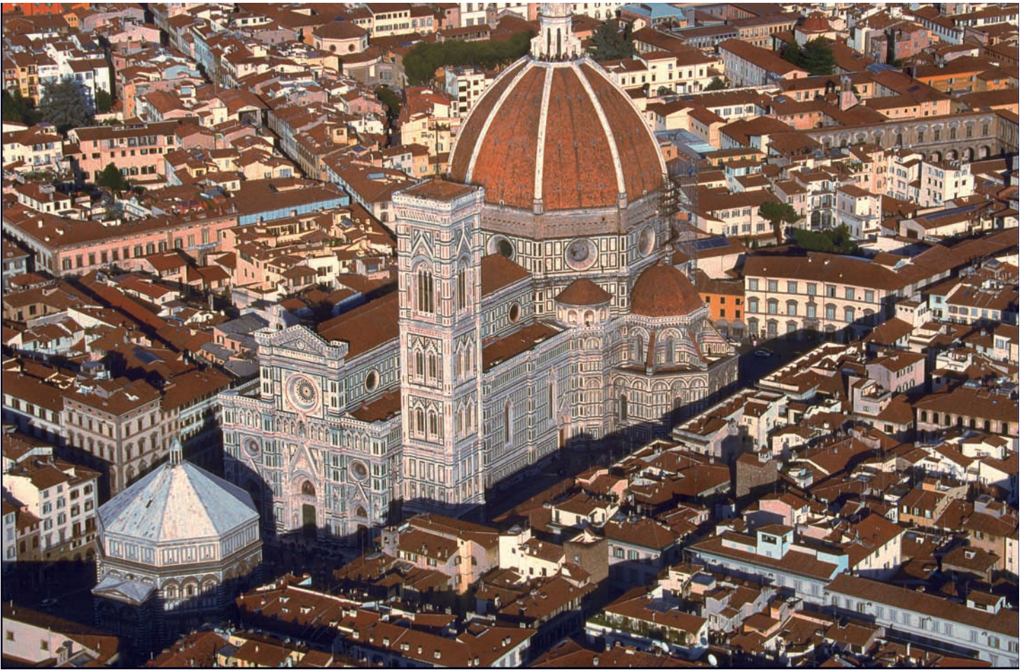
7-36 ARNOLFO DI CAMBIO and others, aerial view of Florence Cathedral (looking northeast), Florence, Italy, begun 1296.
