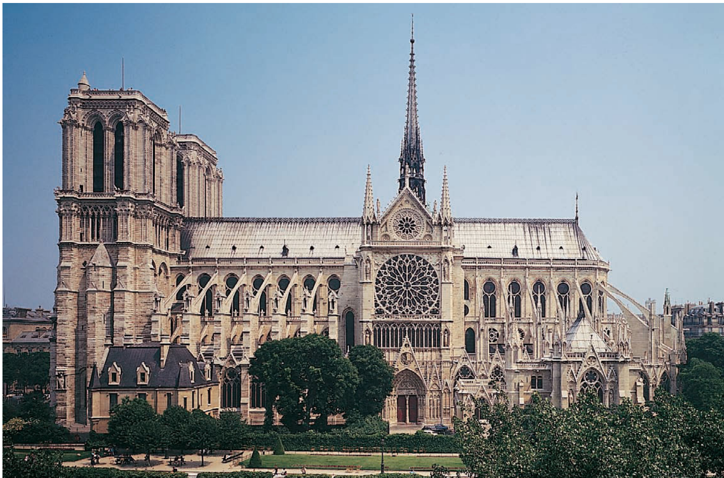
7-8 Notre-Dame (looking north), Paris, France, begun 1163; nave and flying buttresses, ca. 1180–1200; remodeled after 1225.
