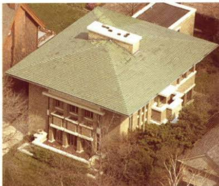
Above and Below: The square plan Bogk residence with its highly ornamental facade of Roman brick.
