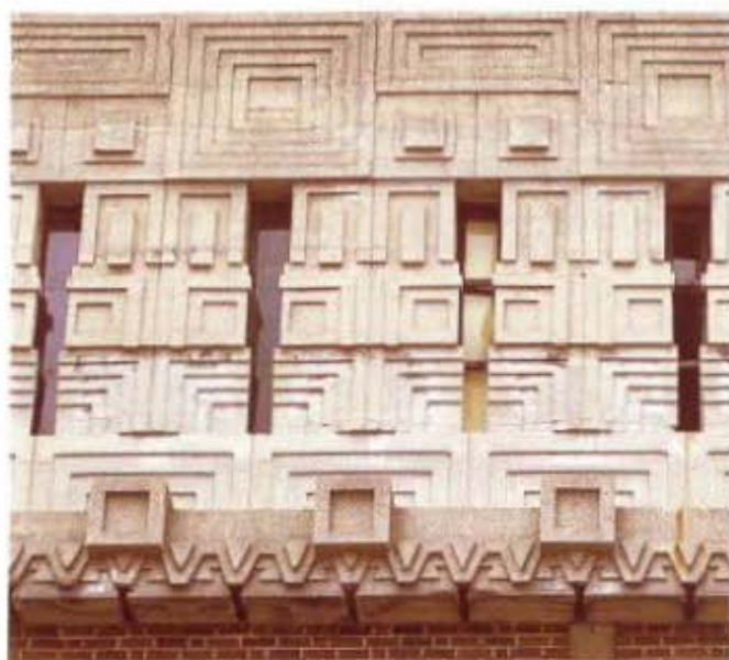
Above and Below: The A.D. German Warehouse. Note the patterned block of the upper story which was designed for cold storage.
