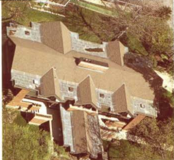
Above and Below: Aerial views of the Beachy house in Oak Park. Constructed of brick and plaster with a wood trim, an earlier house constitutes part of the structure.
