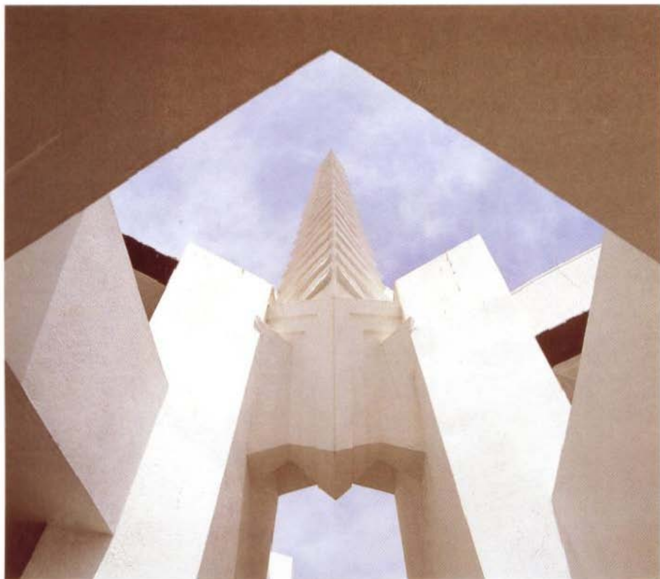
These photographs are of the Anderton Court Shops in fashionable Beverly Hills. The ramp is built to a diamond-shaped parallelogram pattern around the central mast.
