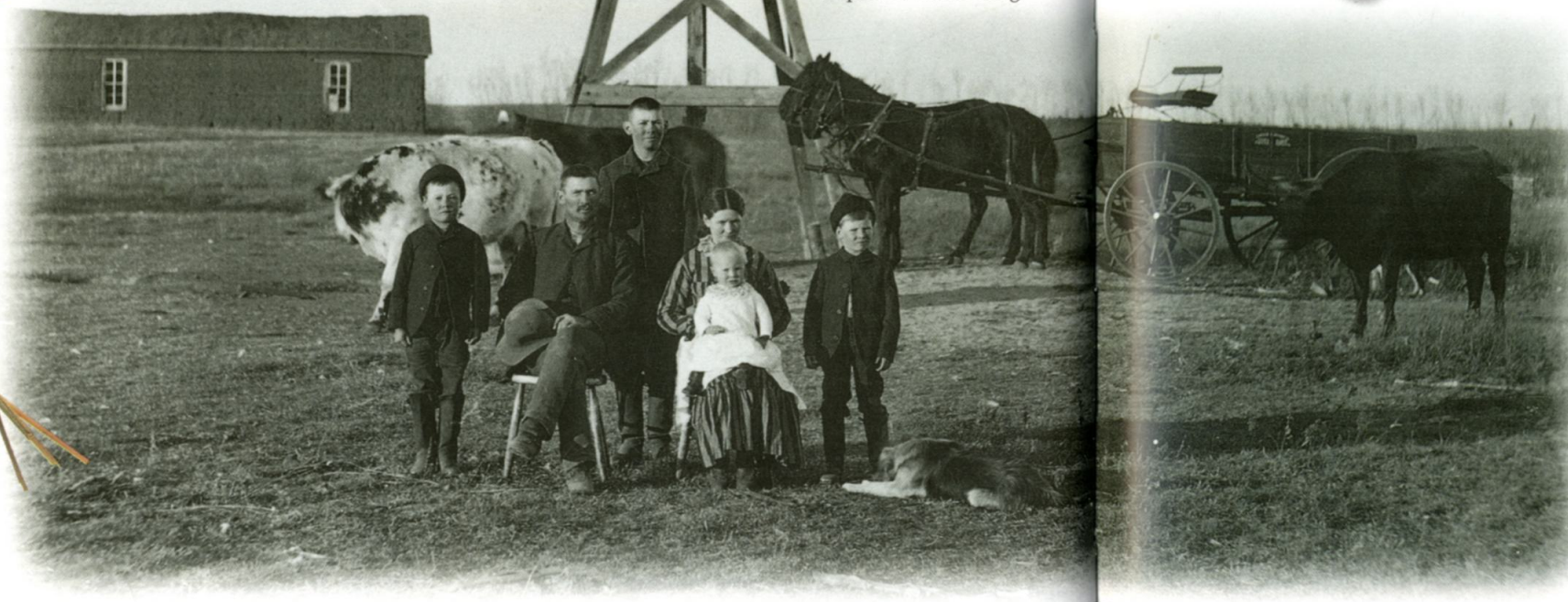
A FAMILY WINDMILL The McCartys of Custer County, Nebraska, gather in front of their wooden windmill, which was essential for pumping water from depths of 200 feet or more. The "tail" of the mill kept it facing the direction of the wind, and also offered a space for advertising.
