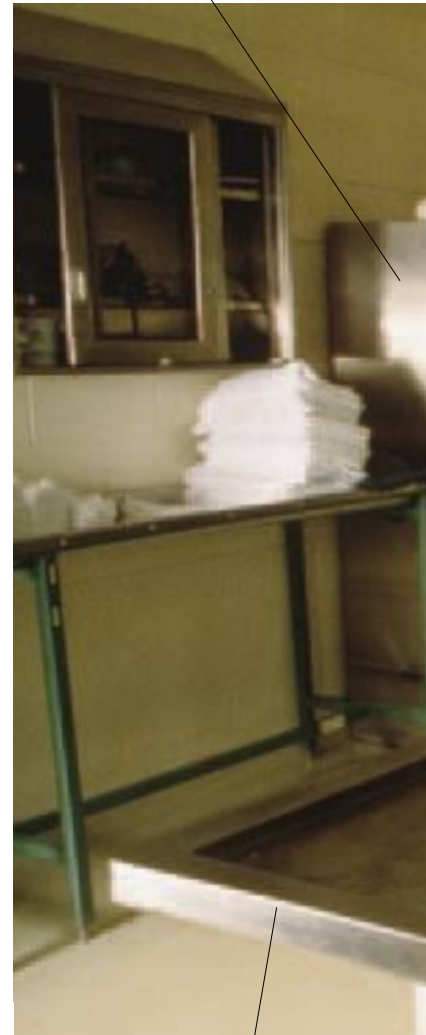
Raised lip prevents liquids from spilling on to floor
