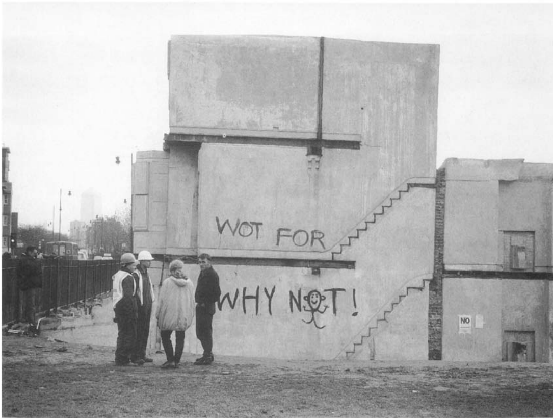
FIGURE 60 House , shortly before demolition
