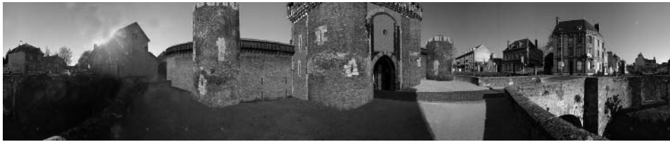
Fig. 4. Created elements: crenellation on top of the bastion towers.
