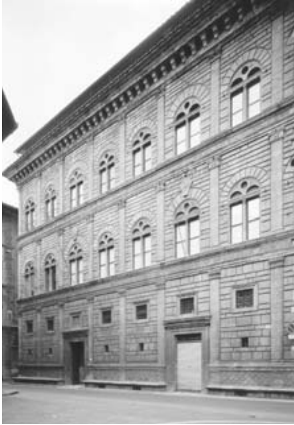
Façade of Palazzo Rucellai, 1455–1470 by Alberti. Palazzo Rucellai, Florence. © Scala/Art Resource, New York.
