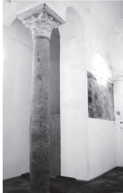
378. Myrelaion, Constantinople. Original marble column and Corinthian capital in the former cistern converted to a chapel
