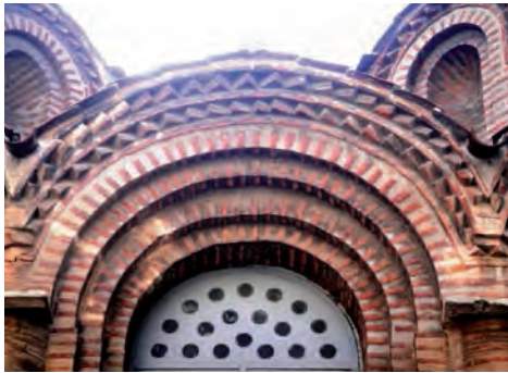
499. Panagia Chalkeon, Thessaloniki. Brick pattern in window arch
