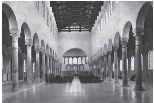
572. San Giovanni Evangelista, Ravenna. Naos looking at bema apse with arcades separating the aisles, clerestory lighting and open roof with exposed wood trusses
