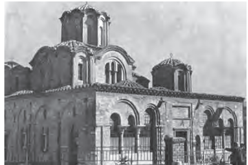
502. Holy Apostles, Thessaloniki. View from the northwest showing central entrance doorway (right) drums of the narthex domes above and the tall drum of the central naos dome (background)
