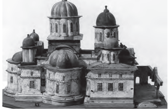
156. Athonite type. Wooden model of the north side of the katholikon , Monastery of Xeropotamou, Mount Athos. Semi-circular apse and square prothesis (left), semi-circular chorostasia (centre left), rectangular liti (centre right) and original narthex portico (right)
