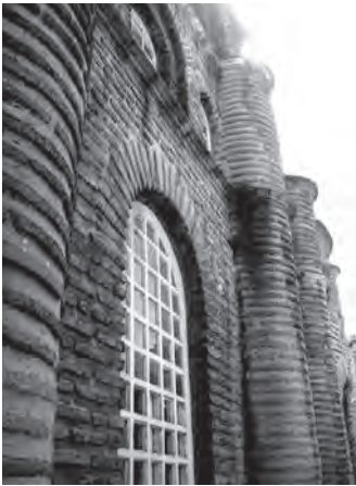
376. Myrelaion, Constantinople. Thin bricks with courses separated by thick mortar joints
