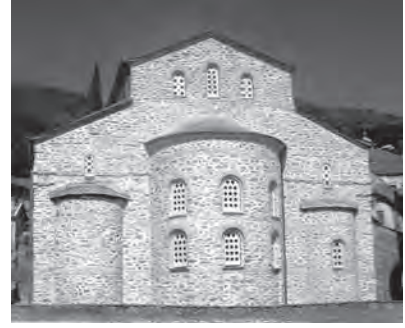
580. Mount Athos, Church of the Protaton. East side with projecting semi-circular apses, the bema in the centre with the pastophoria on either side
