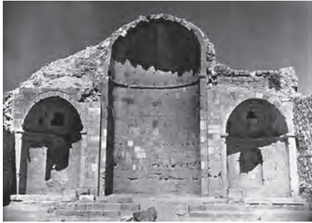
195. Remains of triple semi-circular apses. Sbeitia, Tunisia. Side apses with niches in the exterior semi-circular wall
