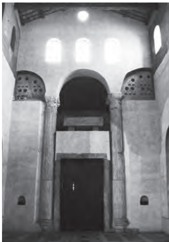
323. Santa Maria in Cosmedin, Rome. Arcade from former church incorporated into the later construction
