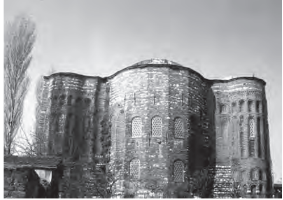
373. St Theodosia, Constantinople. View of polygonal-shaped apses with the larger bema apse in the centre, prothesis (right) and diaconicon (left)
