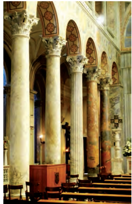
289. Sant'Agnese Fuori le Mura, Rome. Variety of reused Roman marble column shafts
