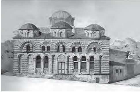
402. St Theodore, Constantinople. Entrance façade with the three narthex domes at the front and the central dome at the back
