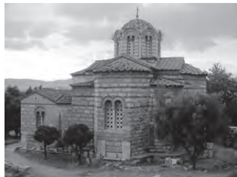
548. Athens, Holy Apostles. In the ancient agora view of the south side with projecting apse (centre), gable roof of the narthex (left), diaconicon and bema apses (right)
