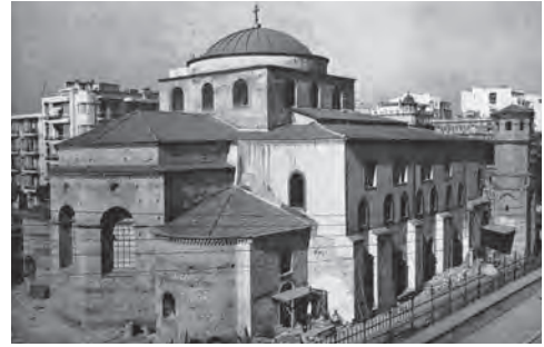
537. Hagia Sophia, Thessaloniki. View from the northeast of prothesis apse (foreground), polygonal shaped bema apse (left) and square drum of central dome
