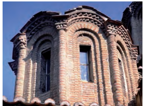
506. Holy Apostles, Thessaloniki. Superb brickwork patterns of a typical drum
