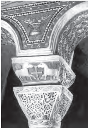
171. Byzantine column capital topped by an 'impost' decorated with a cross supporting arches. San Vitale, Ravenna
