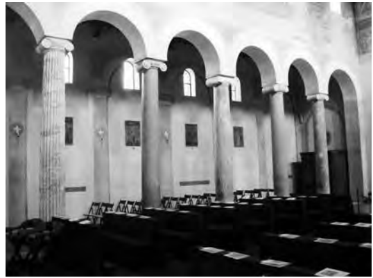
312. San Giovanni a Porta Latina, Rome. Nave arcade with different, reused Roman columns
