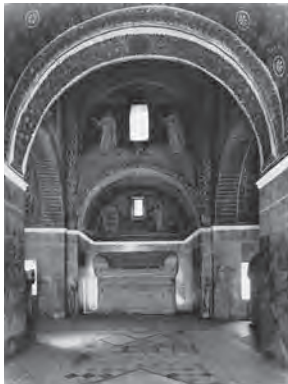
561. Mausoleum of Galla Placidia, Ravenna. Three arms of the cross-in-square visible from the fourth arm
