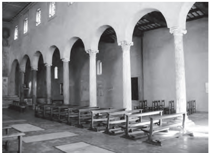
245. San Giorgio in Velabro, Rome. Elegant arcade separating nave from side aisle
