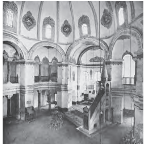
437. SS Sergius and Bacchus, Constantinople. View of former bema apse from the southwest gallery
