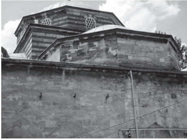
450. St Andrew in Krisei, Constantinople. View from the east of the polygonal shapes of the apse drum (foreground) and central naos drum (background)
