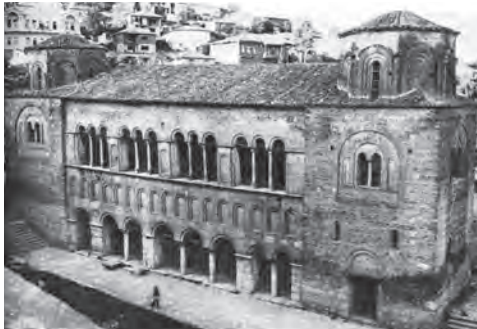
552. Hagia Sophia, Ohrid. Arcaded entrance façade
