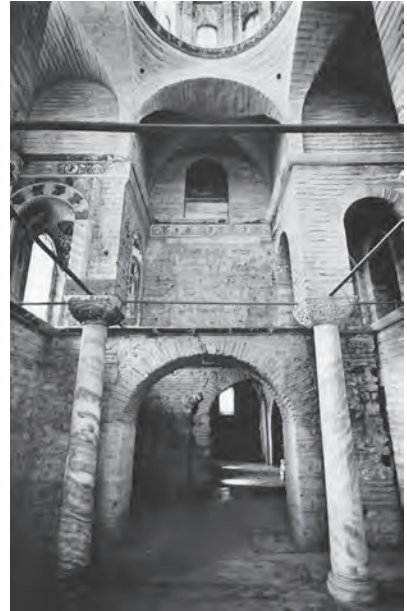
135. Cross-in-square column type – Theotokos Pammakaristos, Constantinople. Interior looking west at narthex entrance
