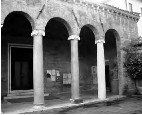
311. San Giovanni a Porta Latina, Rome. Entrance portico with reused, ancient columns of different lengths
