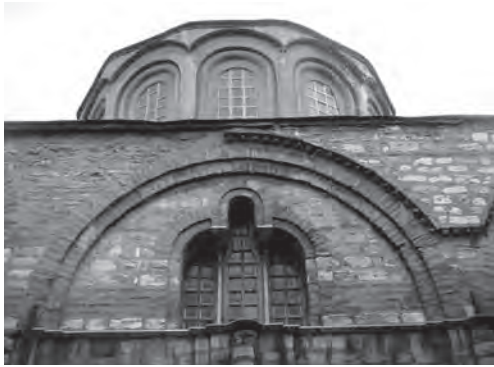
447. St Saviour in Chora, Constantinople. Striking triple window and arched drum at east end of parekklesion
