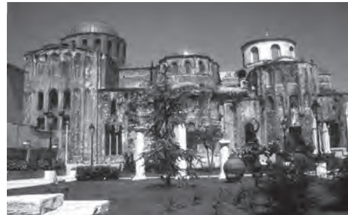
425. St Saviour Pantokrator, Constantinople. View from the east showing the three apses and reconstructed drum and dome over the north church (right)
