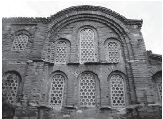
400. St Saviour Pantepoptes, Constantinople. Close-up of the arched windows in the southern arm of the cross-in-square plan
