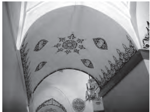
453. St Andrew in Krisei, Constantinople. Barrel vault over side space with Ottoman decoration
