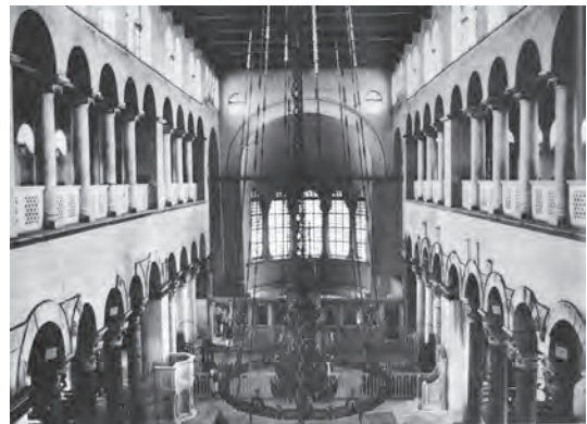
199. Galleries of St Demetrios, Thessaloniki. Separation from naos space by small arcade on either side
