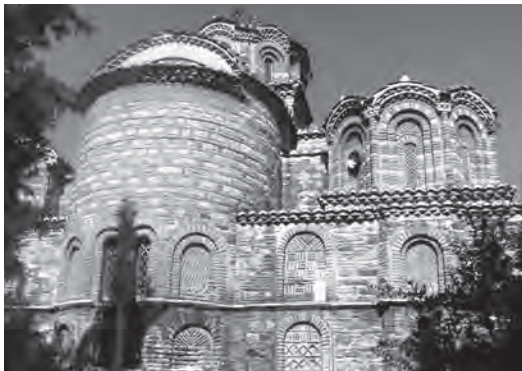
526. St Catherine, Thessaloniki. East end with projecting semi-circular bema apse (left) and polygonal drum of the prothesis dome (right)
