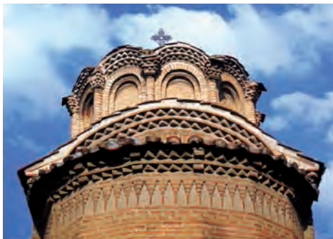
507. Holy Apostles, Thessaloniki. Superlative brickwork at the top of the of the semi-circular bema apse and top of the drum of the central naos dome
