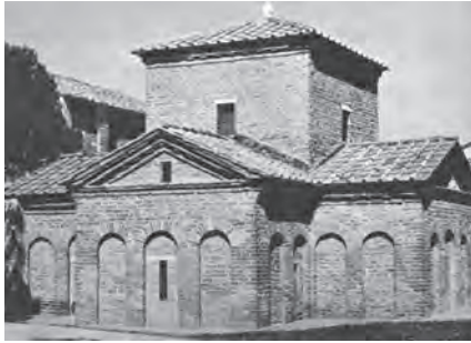
559. Mausoleum of Galla Placidia, Ravenna. Clear view of cross-in-square form (apse in foreground)
