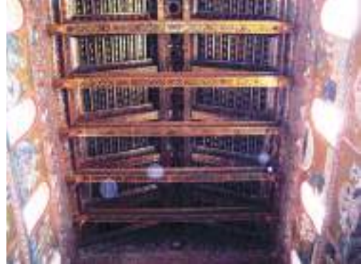
1096. Cathedral, Monreale. Interior view of the decorated roof trusses and underside of the tiles
