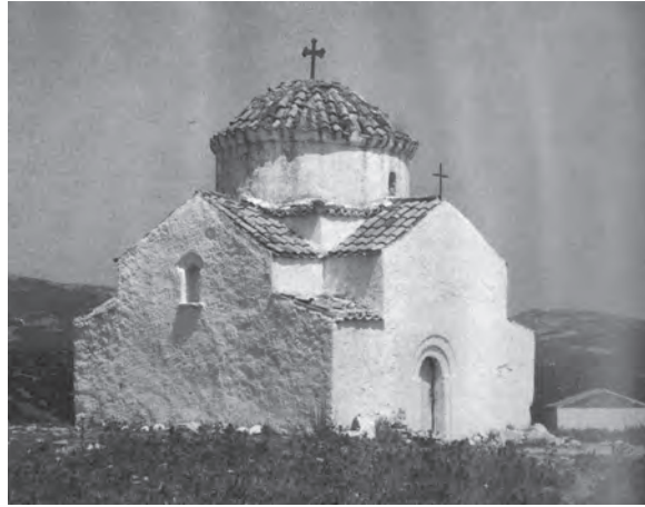
132. Typical cross-in-square church, Greece. Dome covered with tiles and arms of the cross with gable roofs
