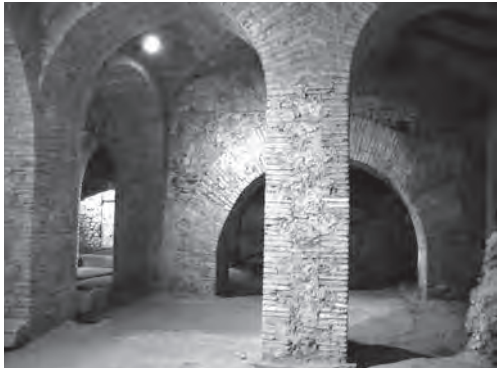
256. San Crisogono, Rome. Extensive arch support system in the original basilica
