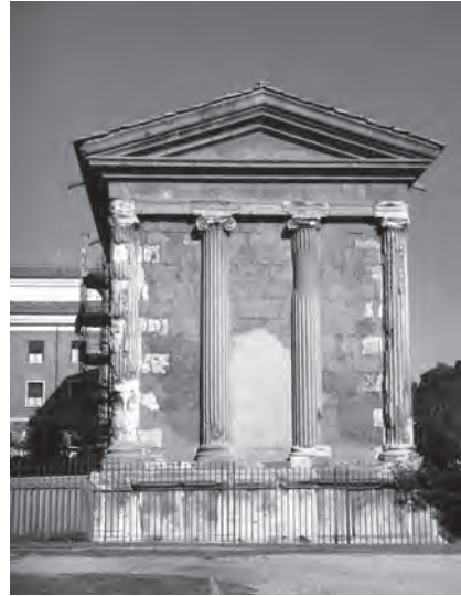
258. Santa Maria Egiziaca, Rome. Walls built between the columns of the Roman temple form an enclosed space for the sanctuary
