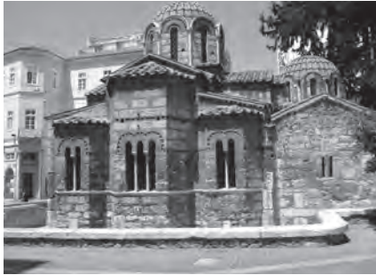
545. Athens, Panagia Kapnikarea. View from the south with naos dome (centre), bema apse dome (right) and visible sunken entrance level (left)
