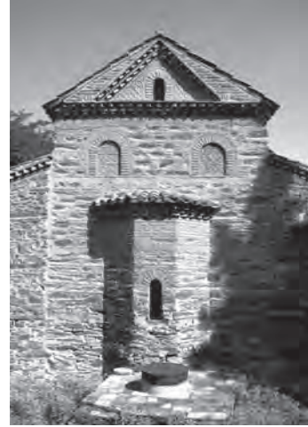
495. St Nicholas Orphanos, Thessaloniki. View from the east of small naos and projecting bema apse
