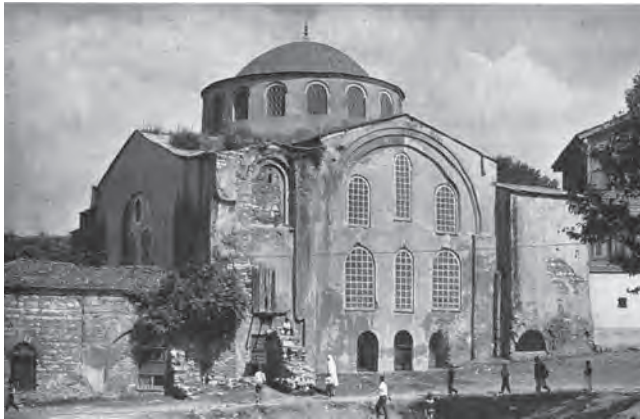
413. Theotokos Kyriotissa, Constantinople. View from the southwest showing the clear cross-in-square form along with cylindrical drum, its arched windows and the dome
