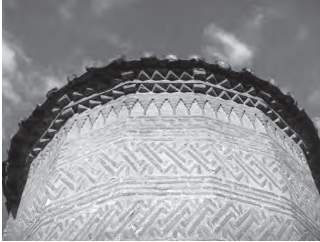
509. Holy Apostles, Thessaloniki. Detail of intricate brick pattern in the bema apse
