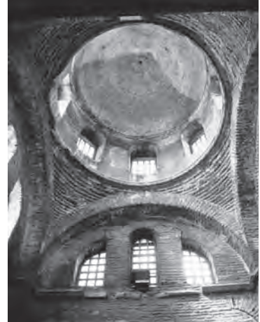
386. Theotokos Panachrantos, Constantinople. Dome, drum, pendentives and supporting arches
