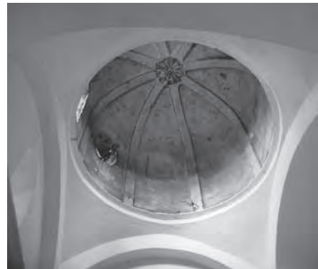
411. St Theodore, Constantinople. A narthex dome with some windows in drum blocked
