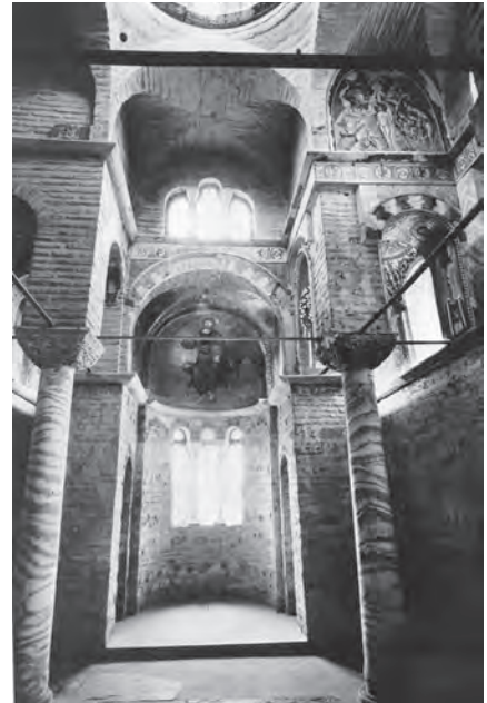
133. Cross-in-square column type – Theotokos Pammakaristos, Constantinople. Interior looking east at apse
