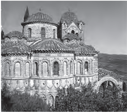
625. Mystras, Pantanassa. East side with projecting apses of bema (centre) and pastophoria on either side
