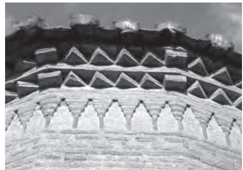
508. Holy Apostles, Thessaloniki. Detail of the brick pattern at the top of the semi-circular bema apse
