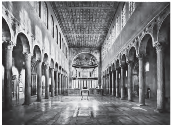
128. Basilica type – Santa Sabina, Rome. Naos looking at apse, arcades with Corinthian columns and wood panel ceiling
