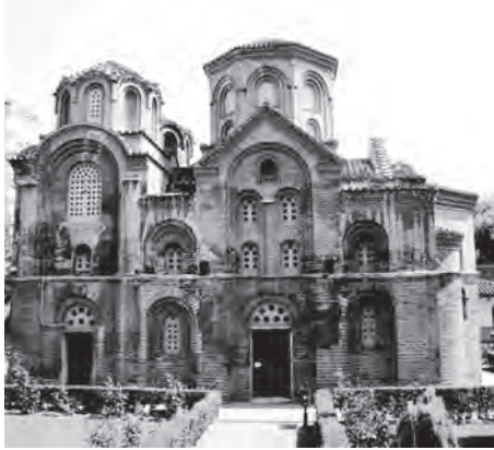
497. Panagia Chalkeon, Thessaloniki. South side with projecting apse (right), polygonal drum of central naos dome (centre) and narthex domes (left)
