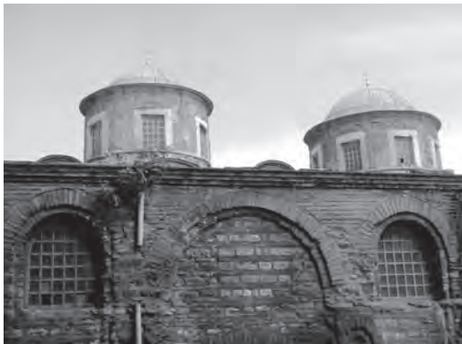
381. Theotokos Panachrantos, Constantinople. Circular cylindrical drums and semi-circular domes of the two churches
