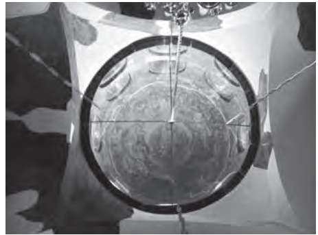
500. Panagia Chalkeon, Thessaloniki. Drum and dome with faint surface decoration
