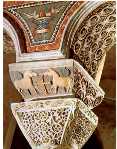
567. San Vitale, Ravenna. Decorative Byzantine column capital and Christian symbols – cross on the 'impost' and doves in the mosaic panel above
