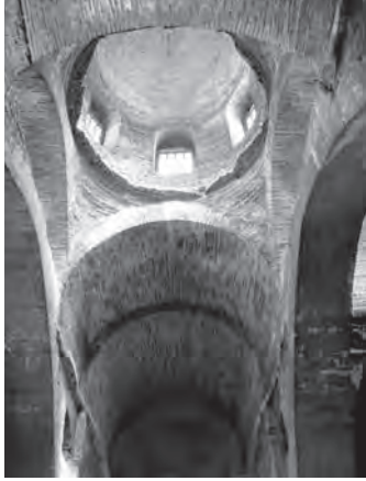
387. Theotokos Panachrantos, Constantinople. Dome (top) and barrel vault (bottom) of the north church
