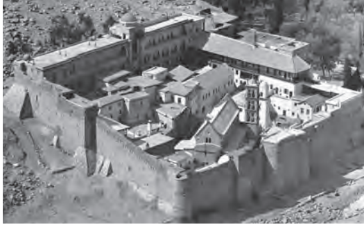
579. Monastery of St Catherine, Sinai. High perimeter wall and katholikon in centre crowded by other buildings
