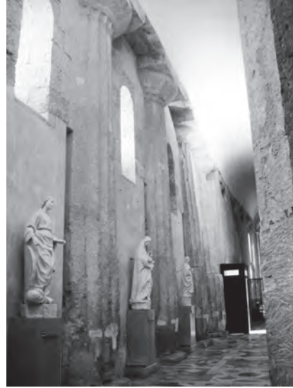
151. Converted type – Duomo Siracusa, Ortegia (former Temple of Athena). Doric columns in the side wall
