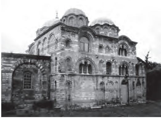
445. St Saviour in Chora, Constantinople. View from the south of narthex (left) and parekklesion (right)
