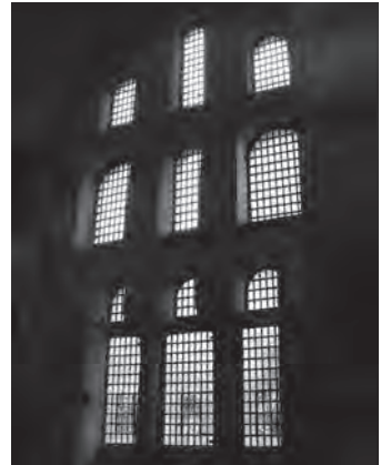
414. Theotokos Kyriotissa, Constantinople. Triple layer of windows lighting up an arm of the cross-in-square
