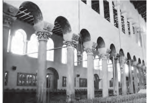
487. Theotokos Acheiropoietos, Thessaloniki. Arcade separating naos from side aisle with marble Corinthian columns and 'imposts' decorated with a cross
