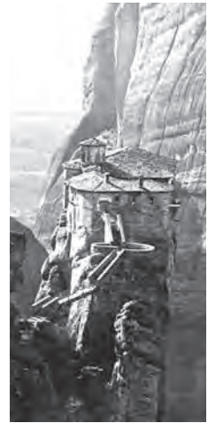
626. Meteora, Roussanou. Spectacular location atop a stone outcrop
