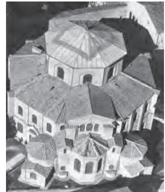
562. San Vitale, Ravenna. Bird's-eye view of centralized form with dominant central dome (top) and smaller domes of the bema and pastophoria apses (bottom)
