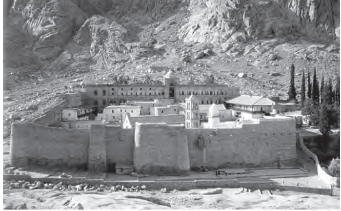
41. Monastery of St Catherine, Sinai. Walled complex with monks' cells forming the rear wall
