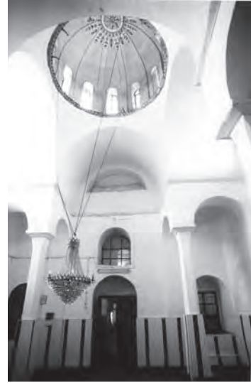
409. St Theodore, Constantinople. Naos dome looking at the entrance from the inner narthex – originally a triple entrance but now the two outer entrances blocked off
