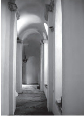
442. SS Sergius and Bacchus, Constantinople. Barrel vault over side passageway
