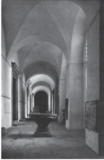
168. Outer narthex, Hagia Sophia, Constantinople. Cross vault ceiling, holy water font, with entrance doors to the inner narthex (left)
