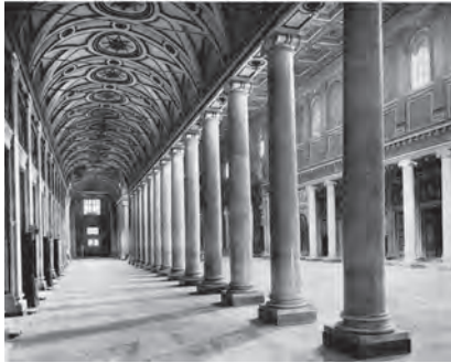
129. Basilica type aisles – Santa Maria Maggiore, Rome. Colonnade with Ionic column capitals and decorated barrel vault
