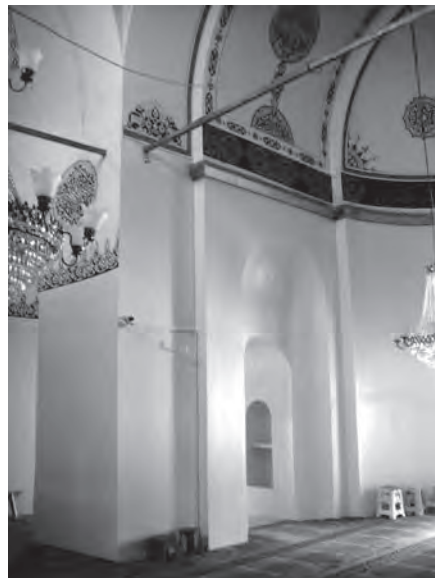
455. St Andrew in Krisei, Constantinople. Former archway into prothesis from bema apse converted into the new entrance to the building
