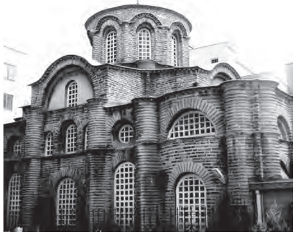
375. Myrelaion, Constantinople. View of the northern side with arched windows piercing the drum of the dome
