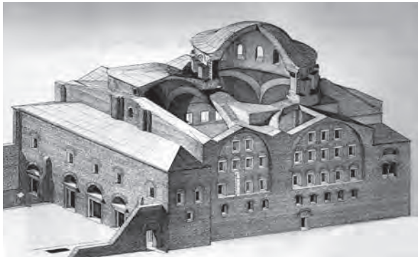
345. Hagia Eirene, Constantinople. Bird's-eye view with the courtyard (left), narthex and cutout viewpoint of the shallow western dome, and central dome over the naos (right)
