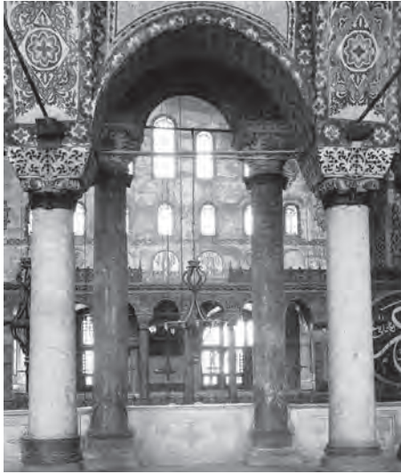
357. Hagia Sophia, Constantinople. Typical decorative arch in the arcade separating naos and aisle
