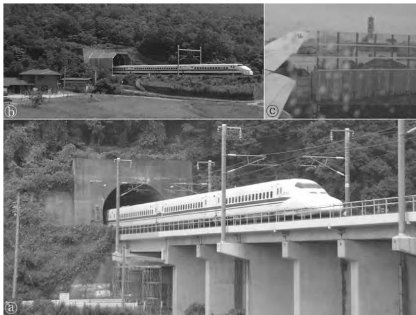
Figure 7.4 (a) A 700-series shinkansen exits a standard tunnel design. (b) A 300-series shinkansen exits a tunnel with a noise-reducing-hood installed. Given the location of the newly constructed house, one can assume the hood has had some positive impact. (c) Noise is clearly not an issue for all in Japan – this house is surrounded by the taxi-ways at Narita Airport.
