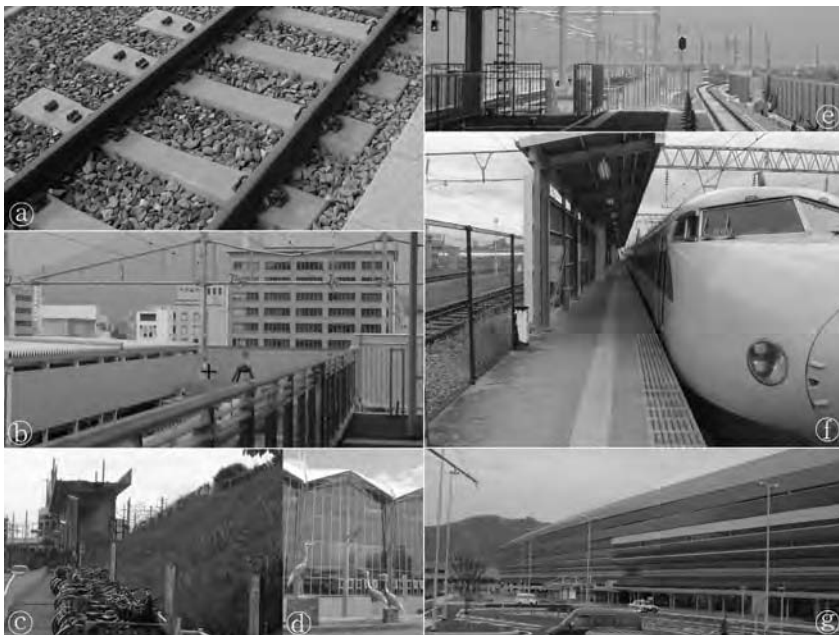
Figure 2.4 (a) On the left is the space where the shinkansen rail will be installed by JR Kyūshū at Shin-Yatsushiro in the future – showing the difference in gauge between the conventional line and the shinkansen line; (b) end of the line at Kagoshima-Chūō with Sakurajima in the distance; (c) a viaduct – to be used by the Kyūshū Shinkansen in the future – near Hakata-Minami station (shinkansen access to which is visible below the viaduct); (d) model cranes on the conventional line platform at Izumi and origami-style cranes in the roof of the shinkansen station; (e) on the right the conventional line curves away from Shin-Yatsushiro to go to join the original Kagoshima Line, on the left the route which shinkansen will take in the future when the Kyūshū Shinkansen is completed; (f) a 0-series-renewal waiting at the narrow Hakata-Minami station – the space to the left will become part of the Kyūshū Shinkansen in the future; (g) the sail-inspired design of Shin-Minamata station.
