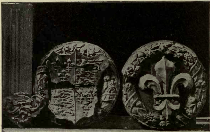
FIG. 203.—Ceiling Bosses from Hampton Court Palace. Sixteenth Century.
