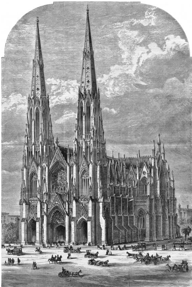
“The largest ecclesiastical edifice in America,” St. Patrick’s Cathedral, New York City, New York, as envisioned in Harper’s Weekly during construction. The building was completed, with some modifications, between 1879 and 1888. From the article “St. Patrick’s Cathedral in New York,” 808, 812.
