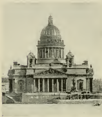
FIG. 207.—ST. ISAAC'S CATHEDRAL, ST. PETERSBURG.
