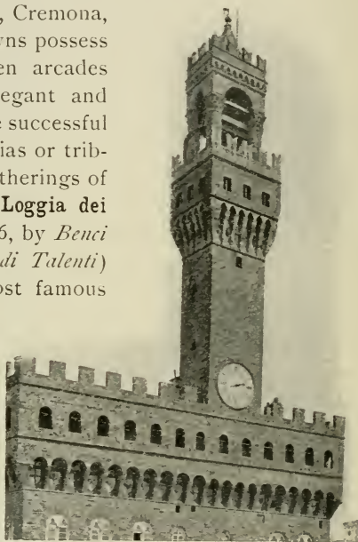
FIG. 155.—UPPER PART OF PALAZZO VECCHIO, FLORENCE.
