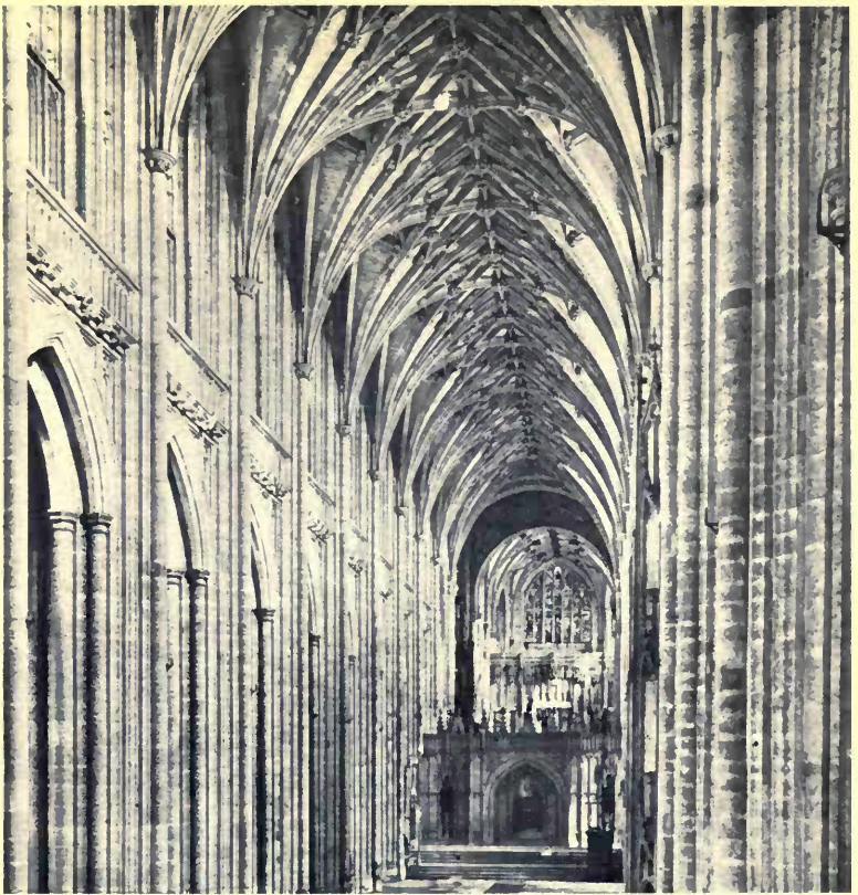
FIG. 304A.—INTERIOR, WINCHESTER CATHEDRAL: LIERNE VAULTING
