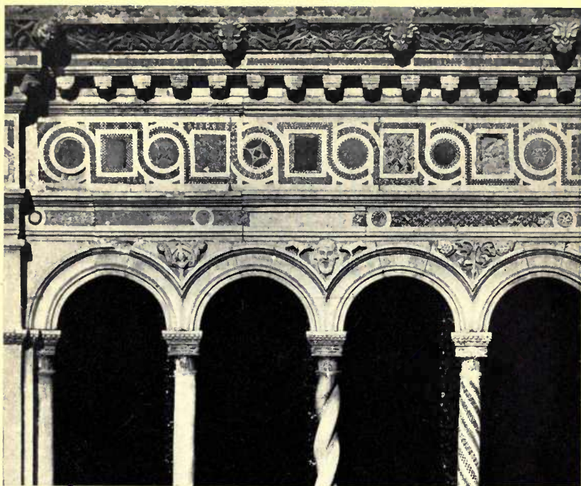
FIG. 214.—DETAIL FROM CLOISTER, ST. JOHN LATERAN
