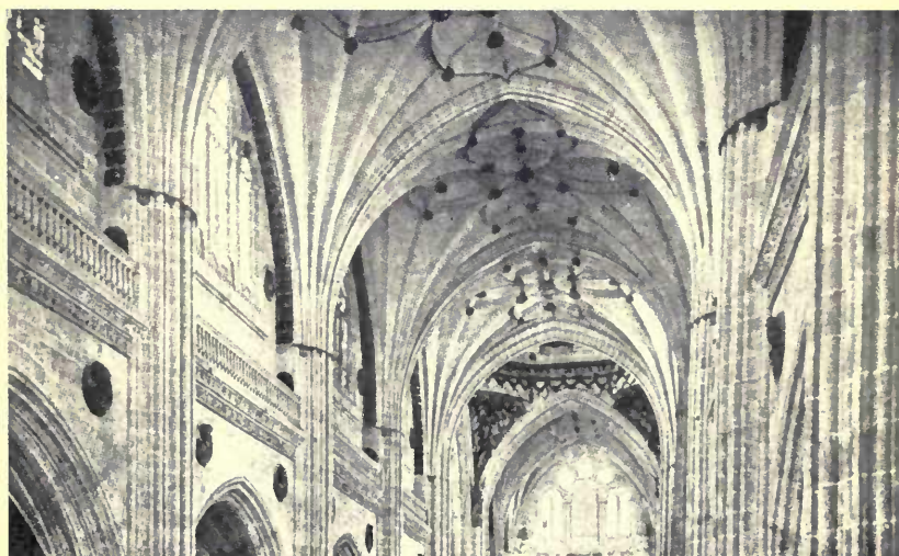
FIG. 383.—VAULTING, CATHEDRAL OF SALAMANCA
