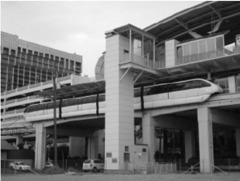
Figure 10-2. Las Vega Monorail Station
