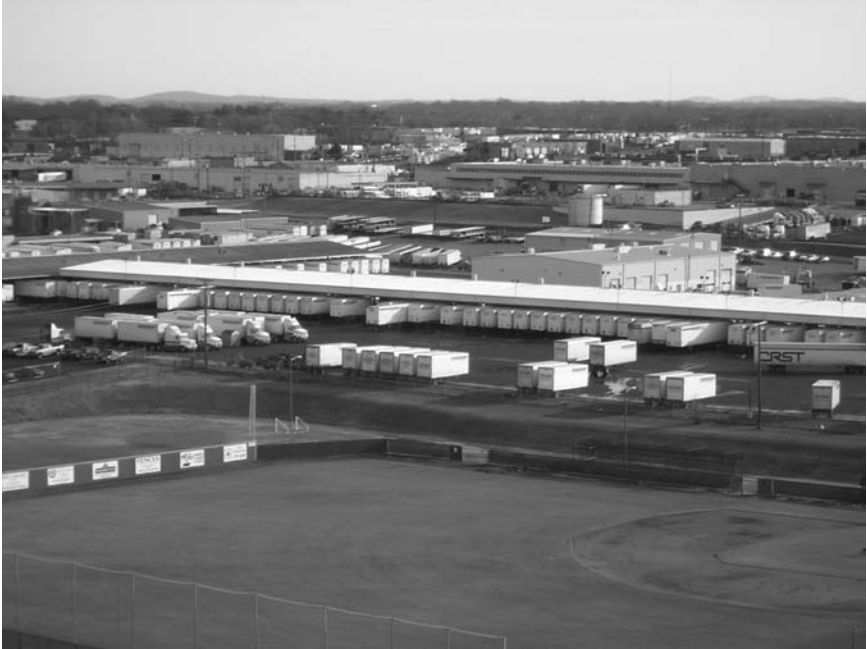
1-5. Trucking Distribution Center in Nashville, TN
