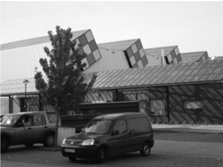
11-4. Rooftop Solar Collector Arrays in Amersfoort, Holland
