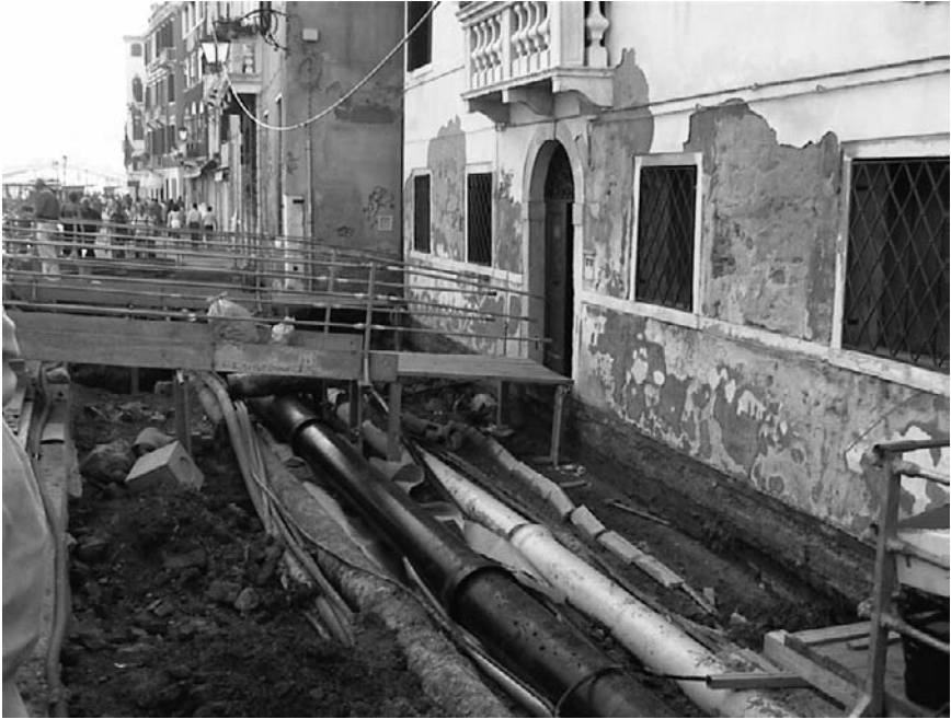
12-9. Installation of Sewage System in Venice
