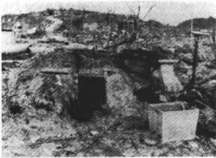
Fig. 1.5. Undamaged earth-covered family shelter in Nagasaki.
