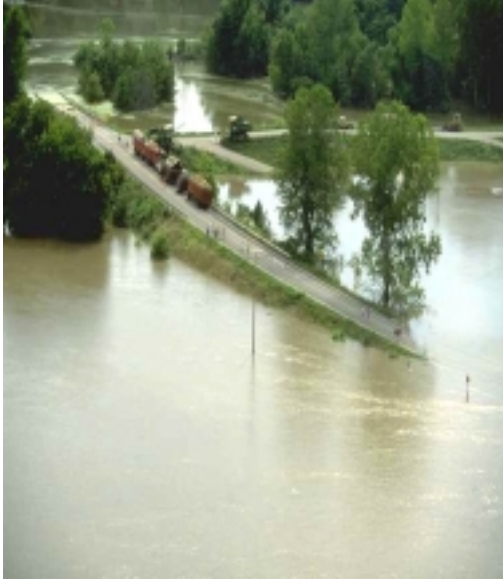
Following a disaster, repairing major roads is a high priority among short-term recovery tasks.
