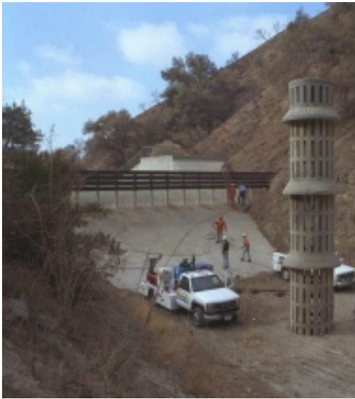
State officials may inspect structures such as dams, levees, and bridges to determine whether repairs are needed.
