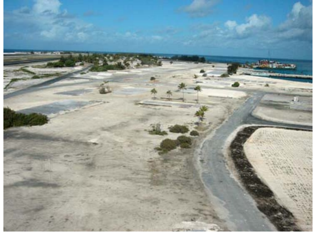
Johnston Atoll after demolition (2004)
