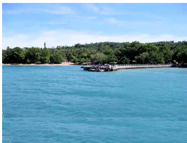
Epi Island—Lamen Bay tender pier
