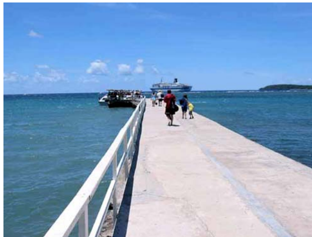
Epi Island—Lamen Bay tender pier
